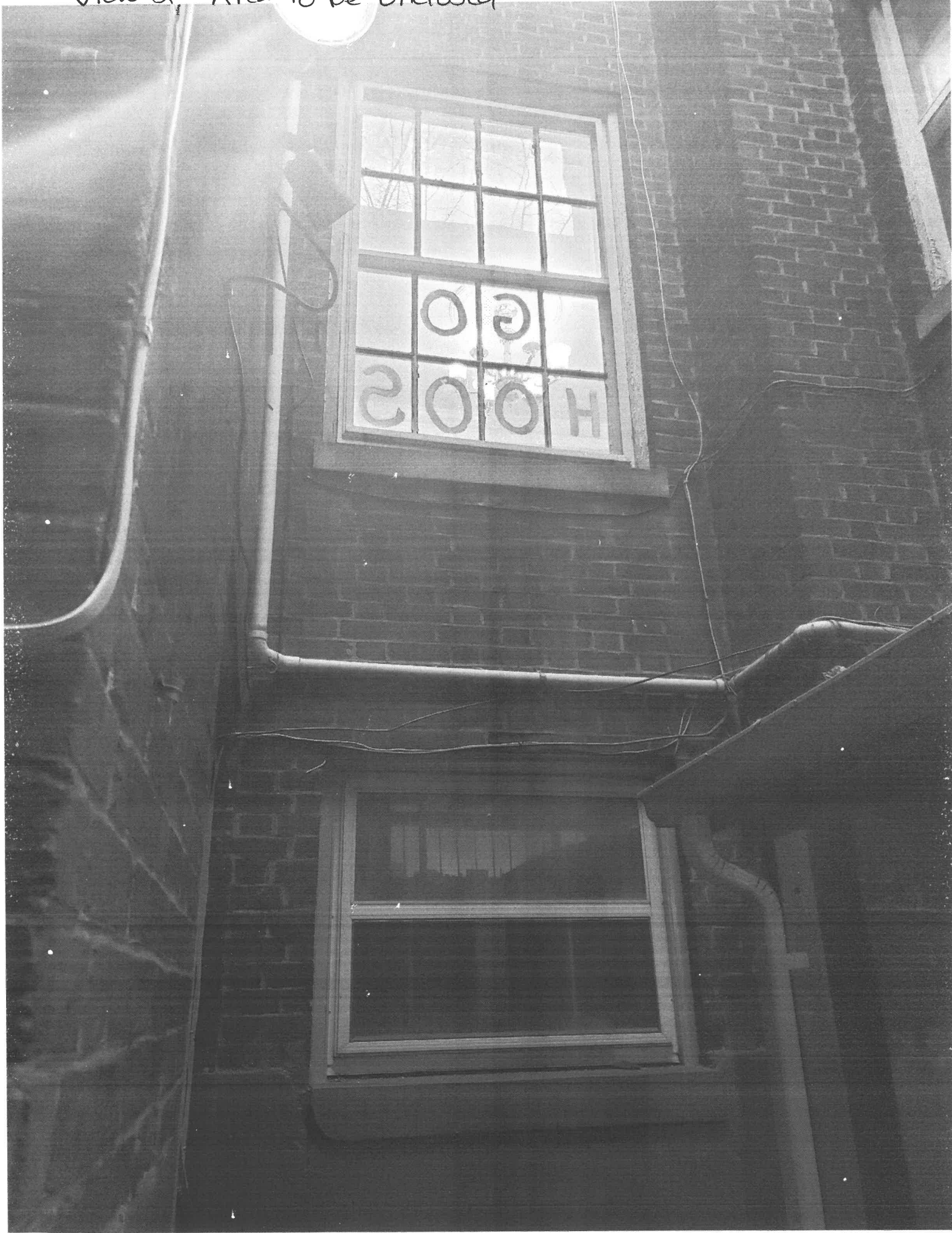
View 2 - Area to be Enclosed
