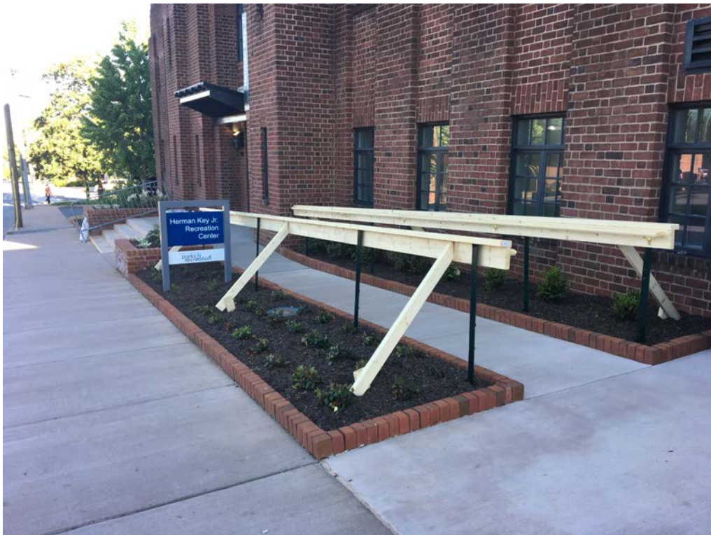
ADA Ramp and Entrance Improvements
