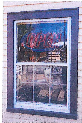
THE UPPER SASH OF THIS WINDOW IS NOT ORIGINAL TO THE BUILDING.
