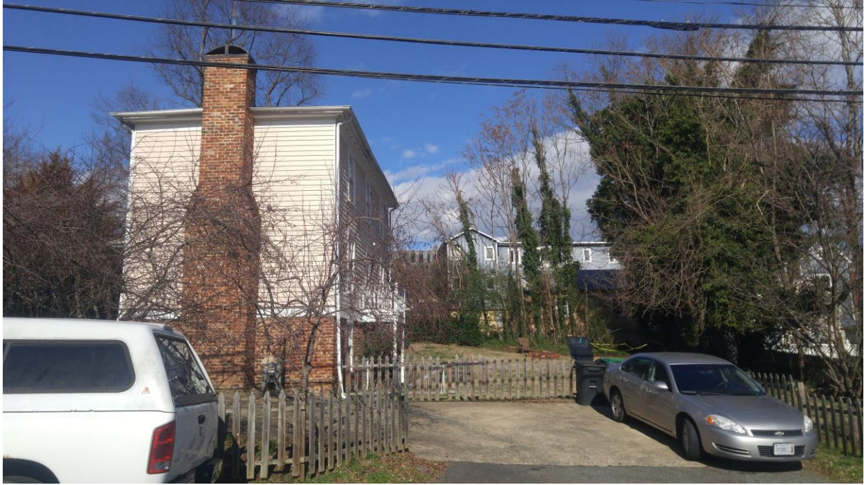
Figure 3: View north towards subject building. Yellow tape marking proposed shed site visible in yard.
