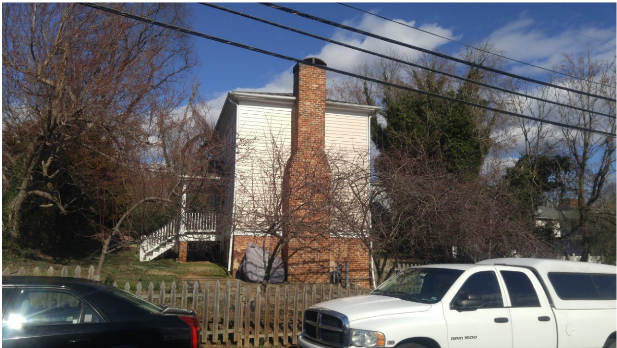
Figure 2: South elevation of subject building.
