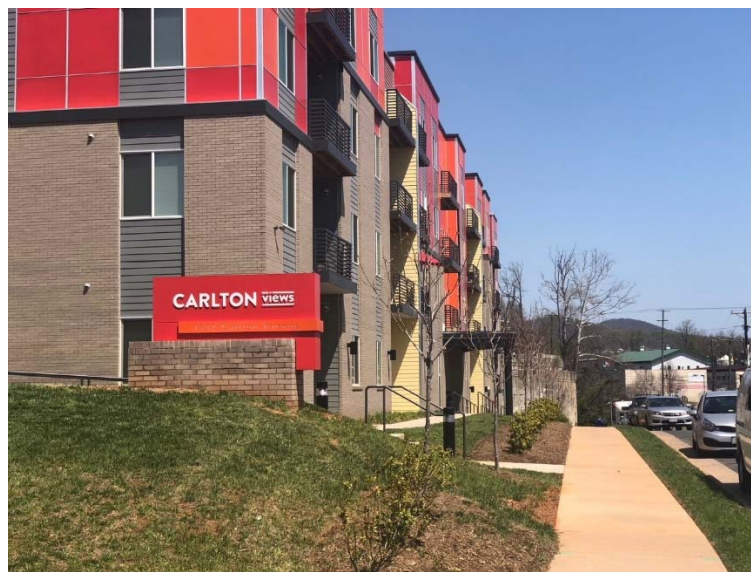
Existing Carlton Views Apartment Building CARLTON VIEWS PUD APPLICATION
