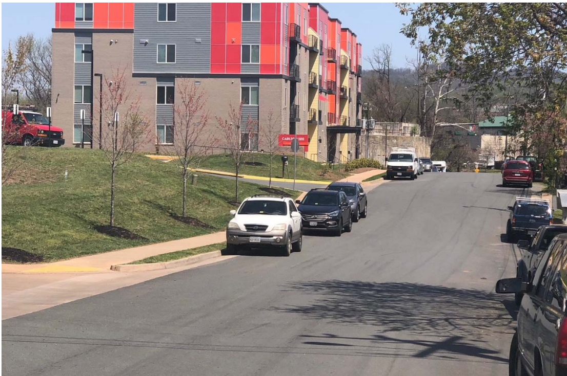
Picture of Carlton Avenue Improvements
