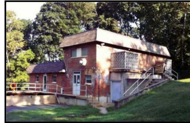
North Rivanna WTP 2 MGD
