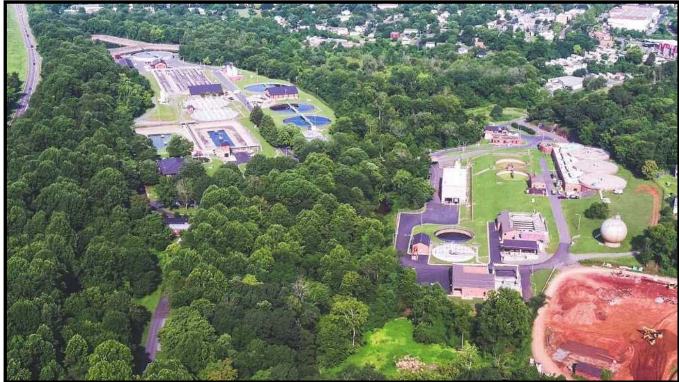
Moores Creek WWTP 15 MGD
