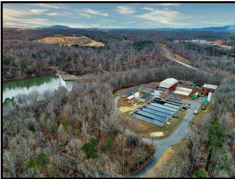
South Rivanna WTP
