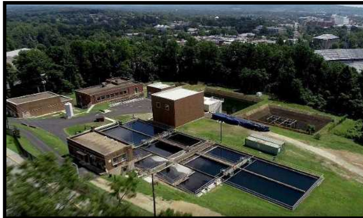
Observatory WTP 7.7 MGD
