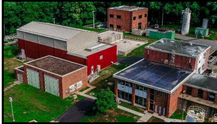
South Rivanna WTP 12 MGD
