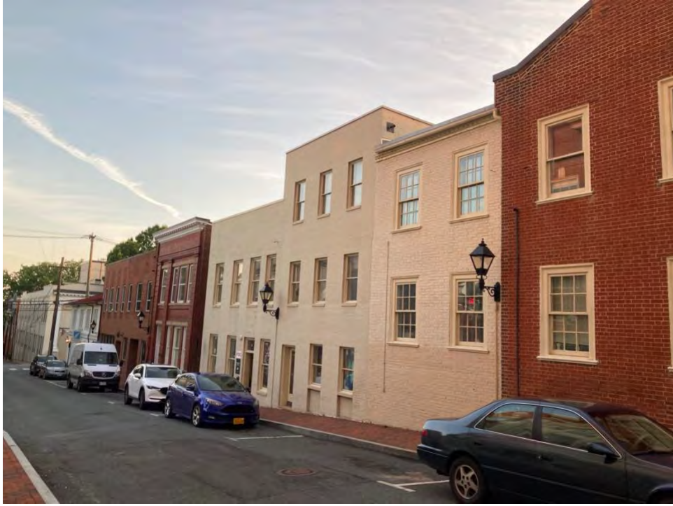
Figure 5: Oblique view of Renaissance School annex buildings along 5 th Street NE, facing southwest.
