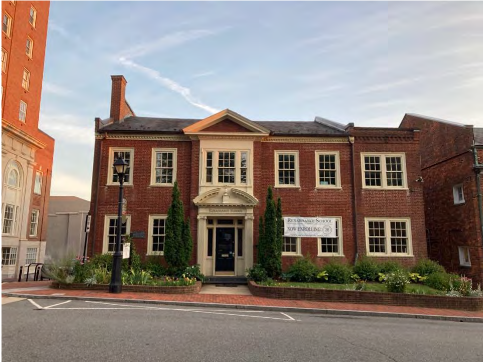
Figure 2: North elevation of 418 East Jefferson Street.
