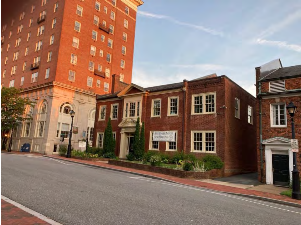
Figure 1: Oblique view of 418 East Jefferson Street, facing southeast
