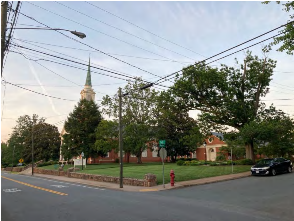
Figure 4: Oblique view of 506 Park Street, facing northeast.
