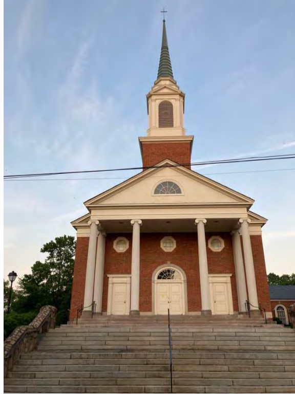
Figure 1: West elevation of 506 Park Street.
