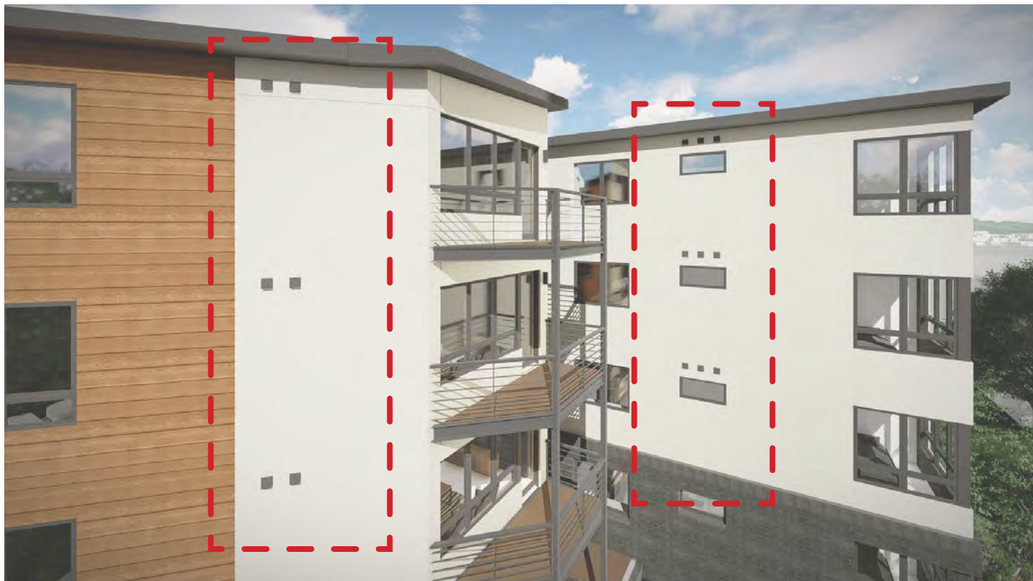
EXHAUST VENTS HAVE BEEN THOUGHTFULLY PLACED AND CONCEALED WHERE POSSIBLE. SEE A4.X SERIES FOR MECHANICAL DIAGRAMS AND 2.X SERIES FOR EXTERIOR ELEVATIONS
