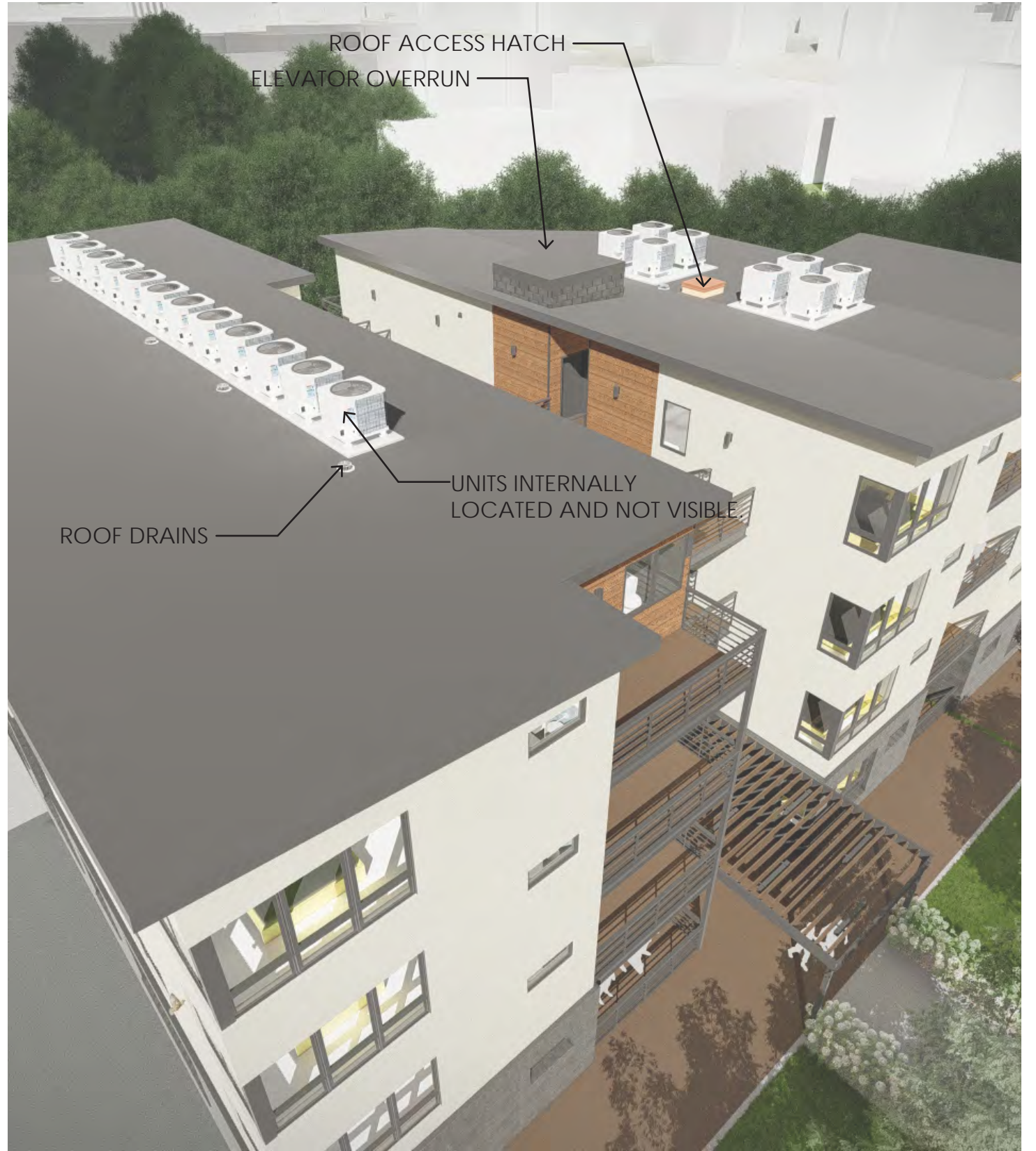
FOR MORE INFORMATION, SEE ROOF PLAN, SHEET A1.5. MECHANICAL EQUIPMENT WILL NOT BE VISIBLE FROM PEDESTRIAN PERSPECTIVE
