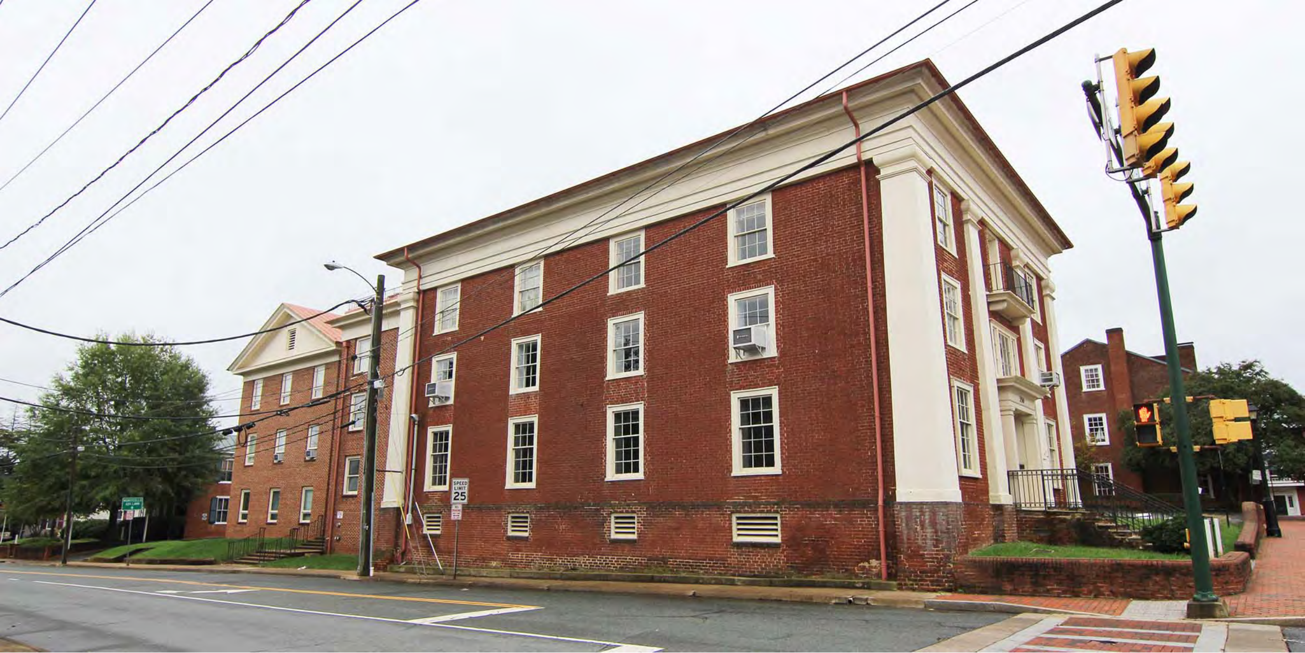
Levy Building: Northwest Corner
