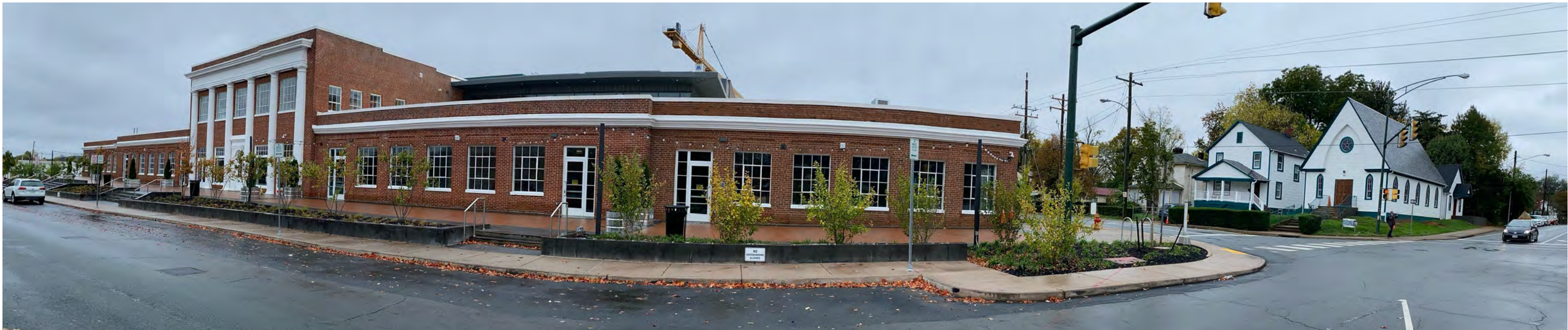
EXISTING GRADY AVENUE FACADE
