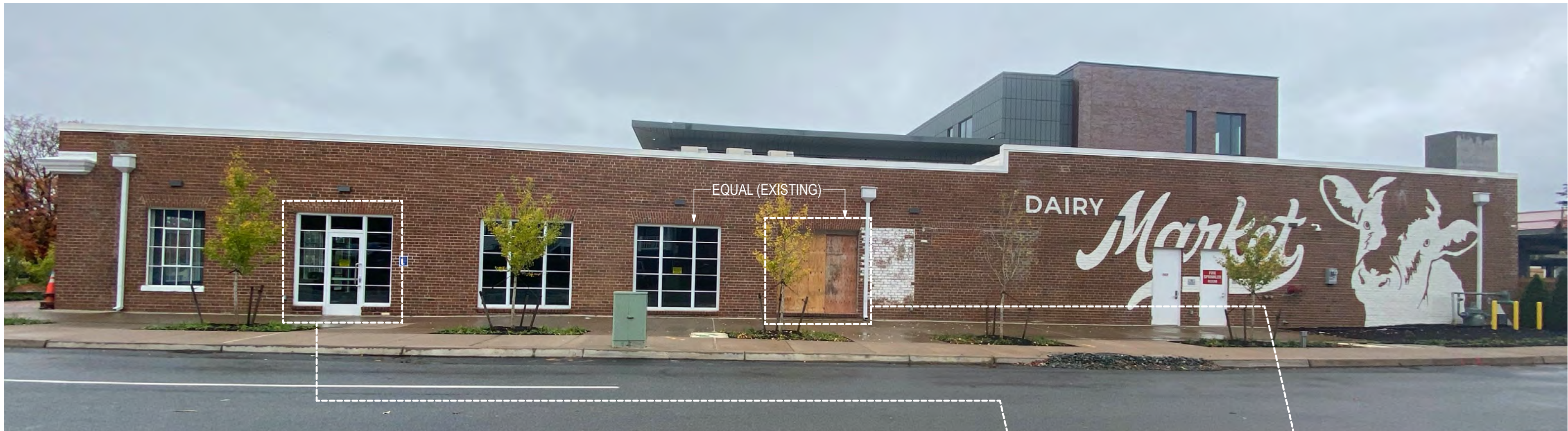
EXISTING GRADY AVENUE FACADE
