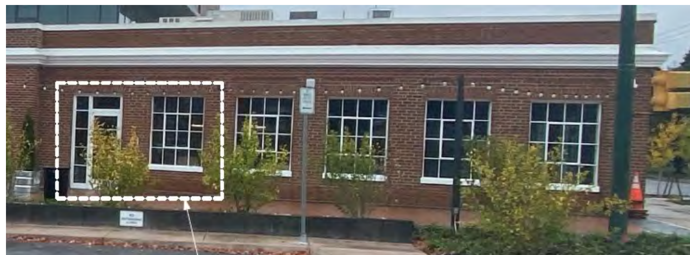
As Built October 2020
