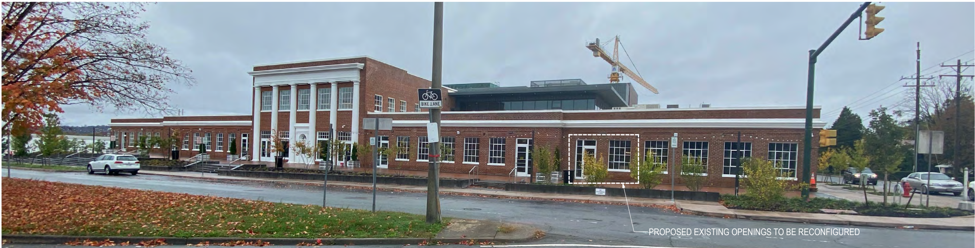
EXISTING GRADY AVENUE FACADE
