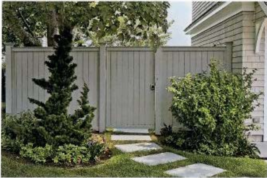
PREFERRED FENCE OPTION: VERTICAL PANEL WOOD FENCE 48"H EXISTING SKIP LAURELS TO STAY ON THE STREET SIDE OF THE FENCE *IN THE EVENT A SKIP LAUREL DIES WE WILL REPLACE IT IMMEDIATELY
