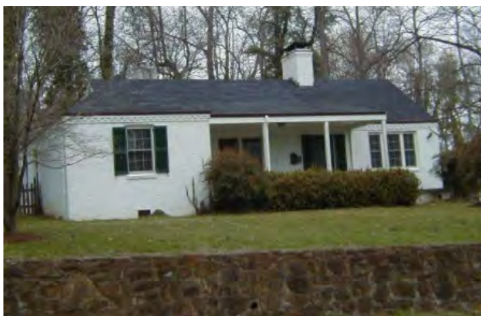
905 (non-contributing, to be razed)
