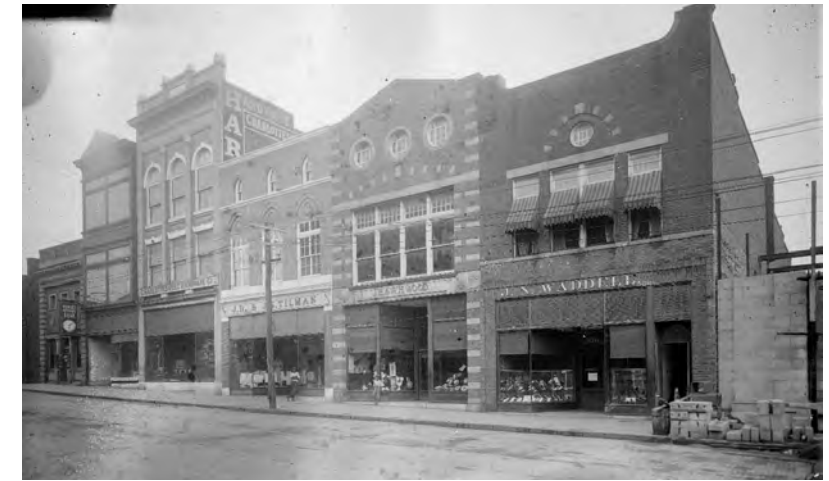
EAST MAIN FACADE, C. 1916
