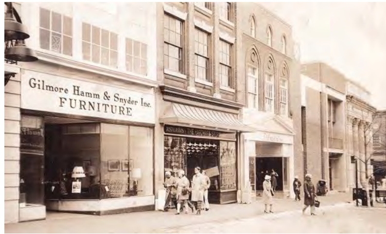
EAST MAIN FACADE, C. 1974
