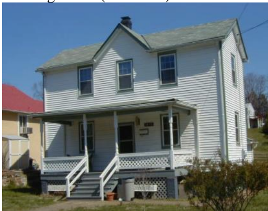
Existing house (to remain)
