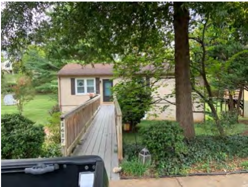
Eastern contiguous house, 1617 East Market Street
