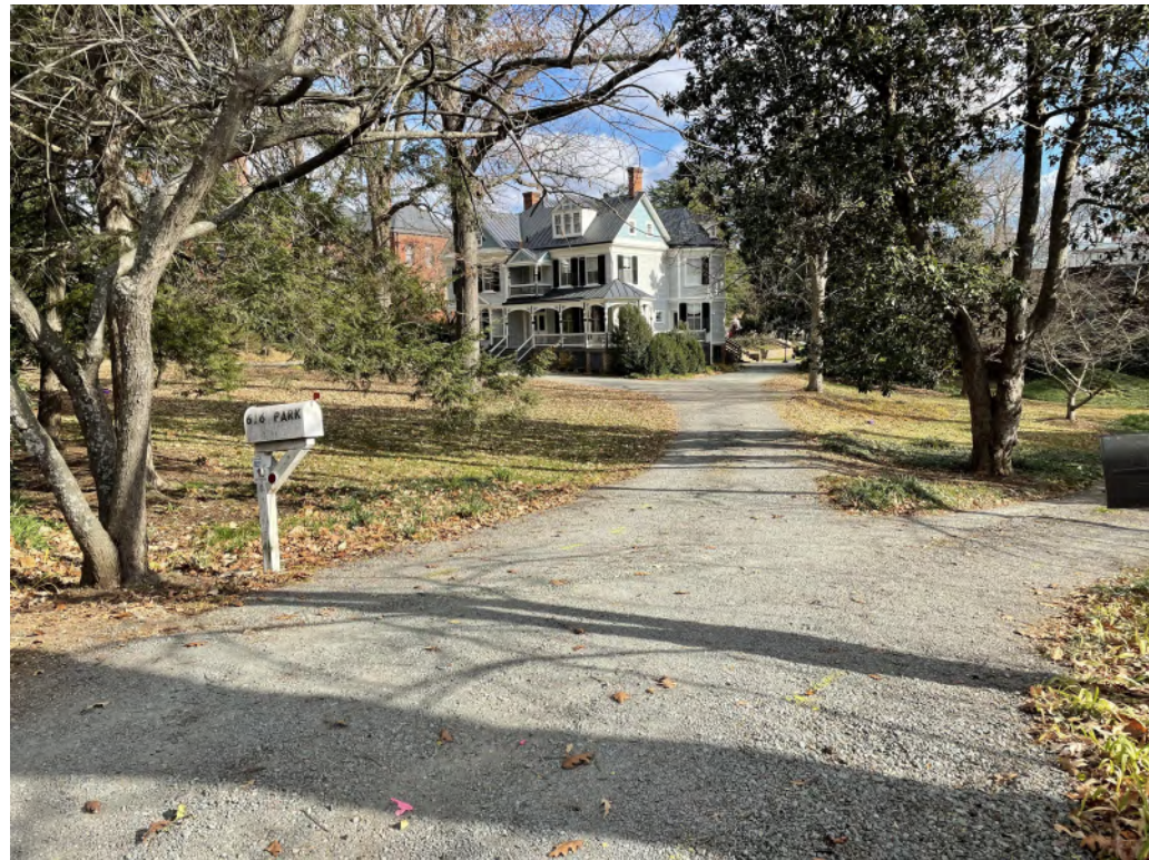
616 Park Street - Southwest View
