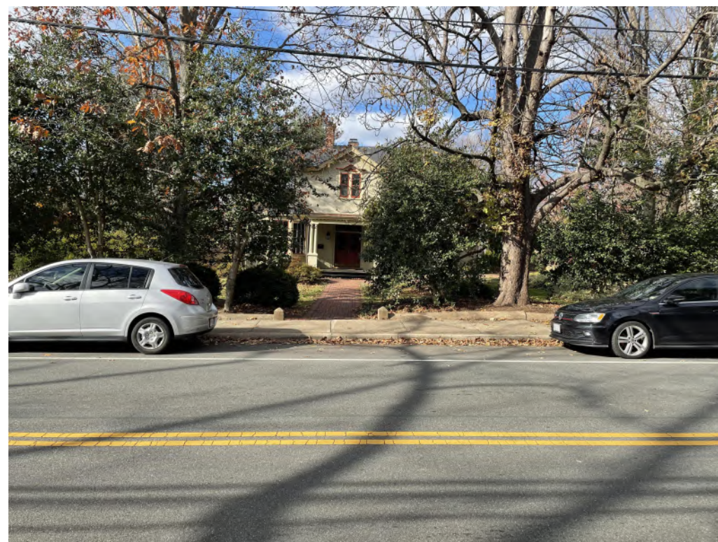
611 Park Street - East/ Park St
