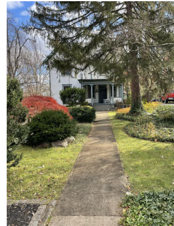
534 Park Street - West/ Park St
