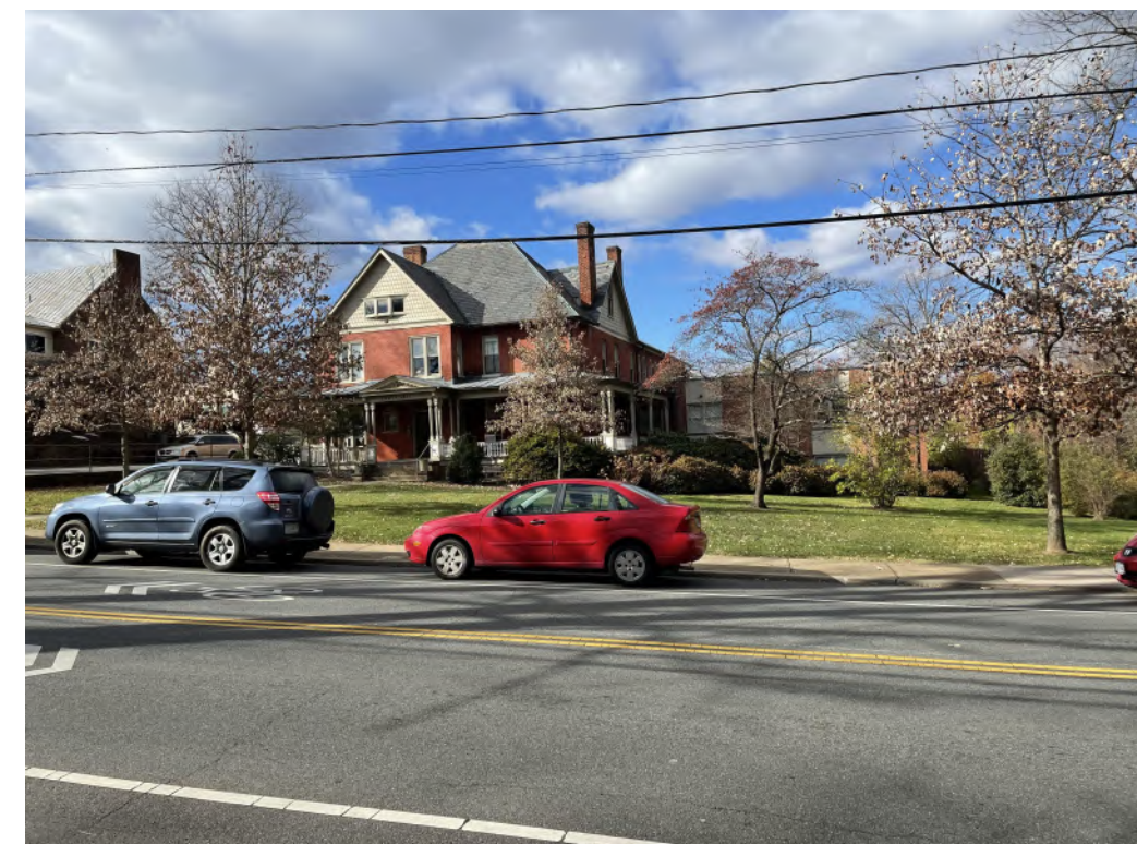
601 Park Street - East/ Park St
