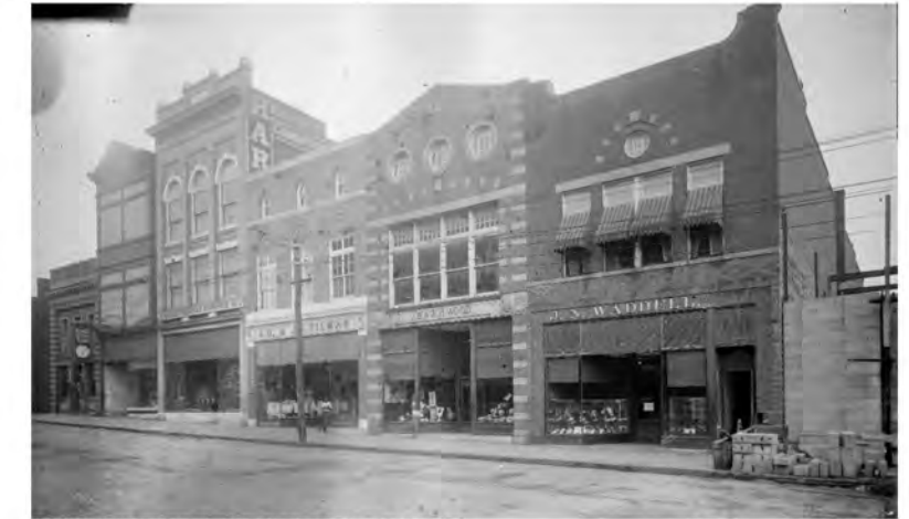
EAST MAIN FACADE, C. 1916
