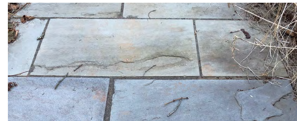
Existing bluestone and stone wall on site
