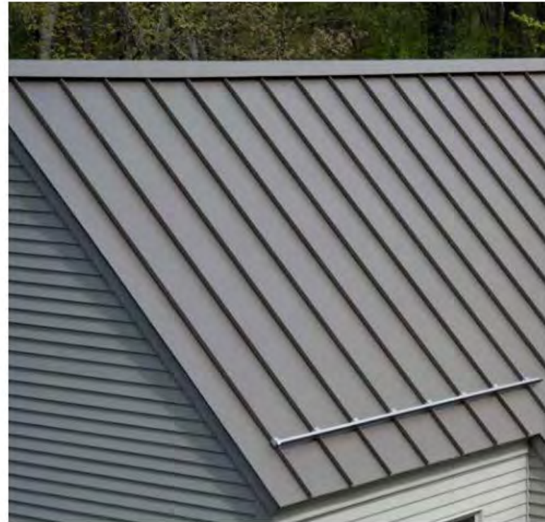
STANDING SEAM ROOF
