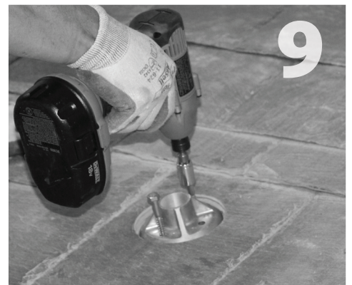
Prior to mounting to the roof, seat the grade-8 cap screw (item 1) through bottom of QBase. Secure the QBase to the rafter with (2) 5/16" lag screws (item 3) and tighten to a snug fit.
