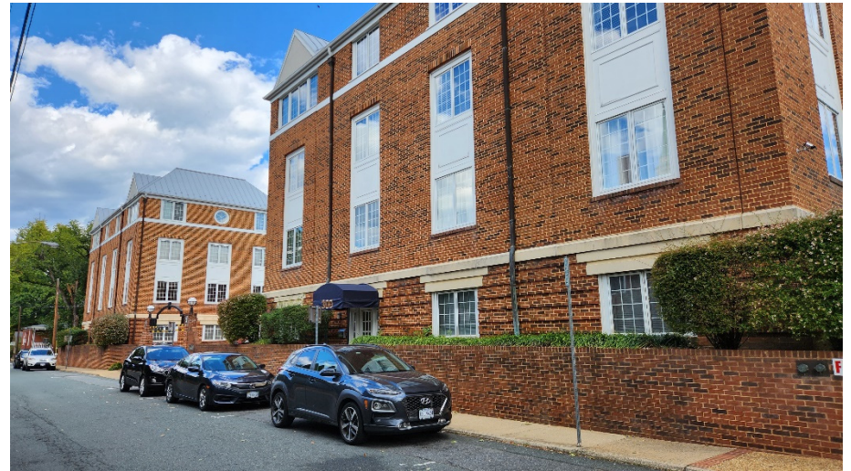
Facing Property from E. Jefferson St./2 nd St. N.E. Intersection
