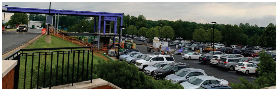
NORTH ELEVATOR AND CROSSWALK
