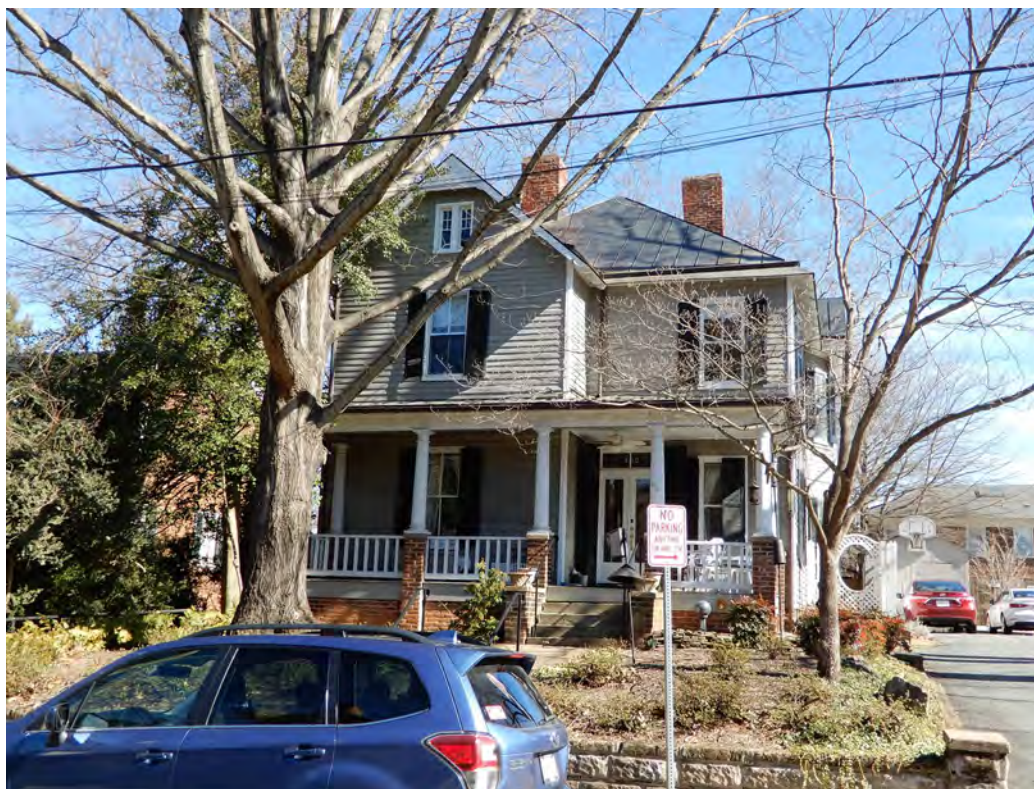
EXISTING WEST (FRONT) FACADE
