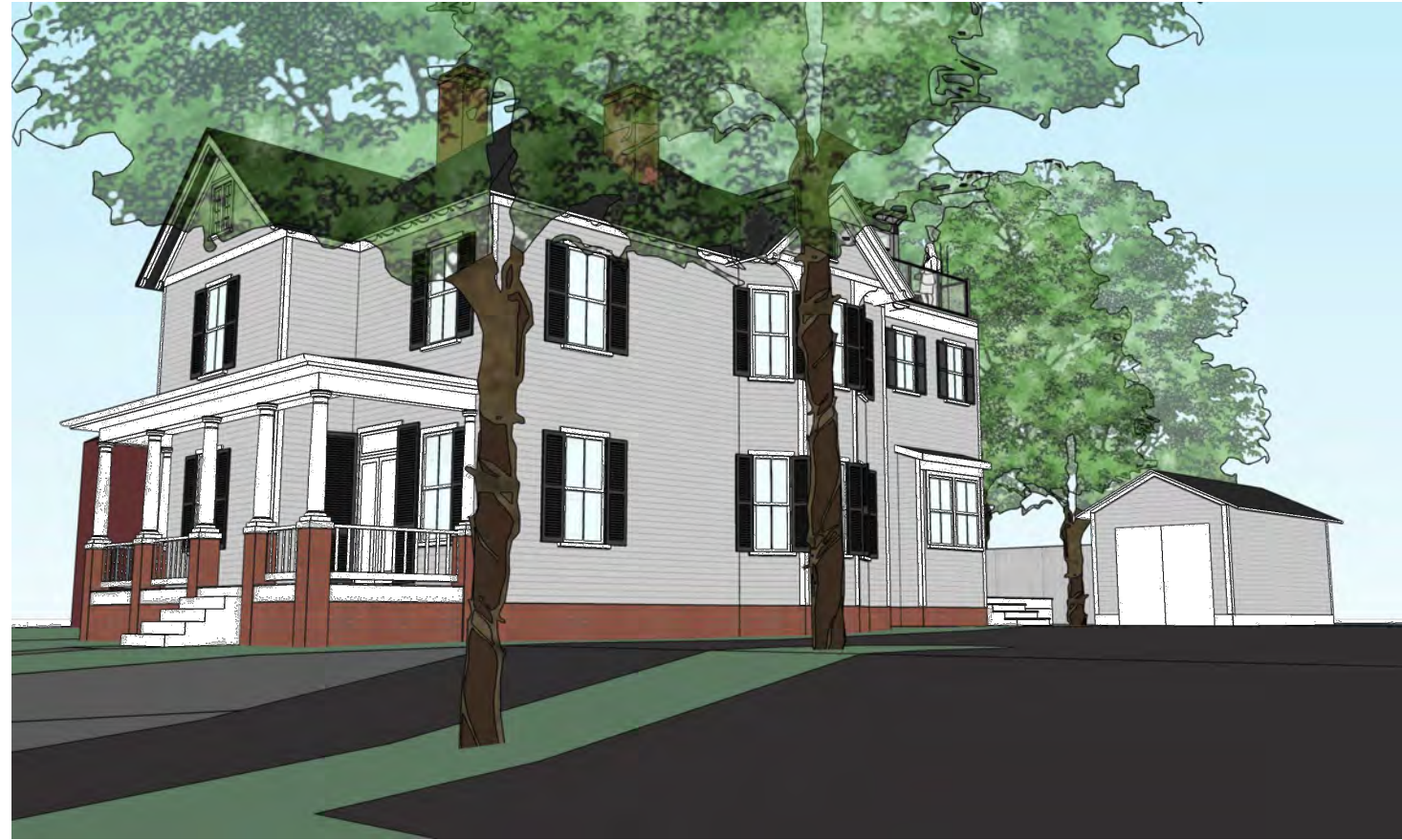
SOUTH VIEW FROM SIDEWALK
