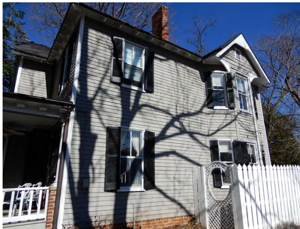
EXISTING SOUTH FACADE
