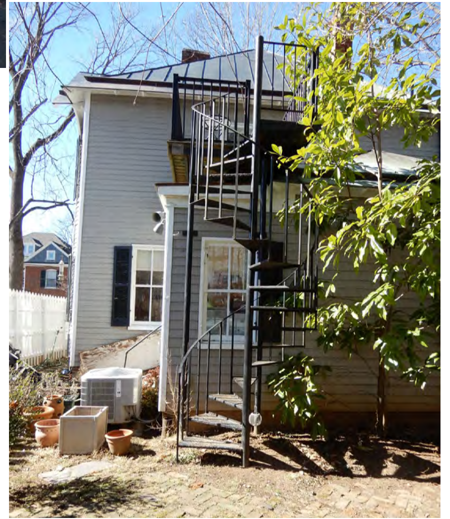
EXISTING EAST FACADE
