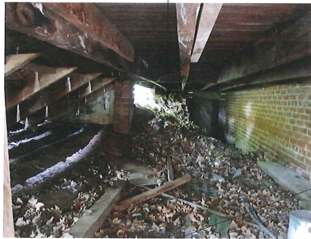
EXISTING COLLAPSED PORCH PIERS AND RETAINING WALL
