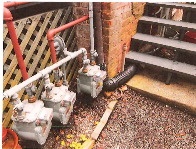
APT. GAS METERS/ EXPOSED DRAINAGE
