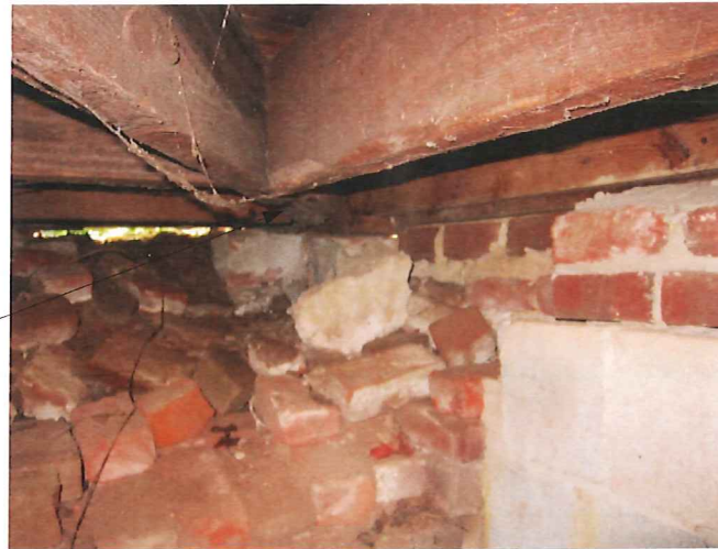
EXISTING COLLAPSED PORCH PIERS AND RETAINING WALL
