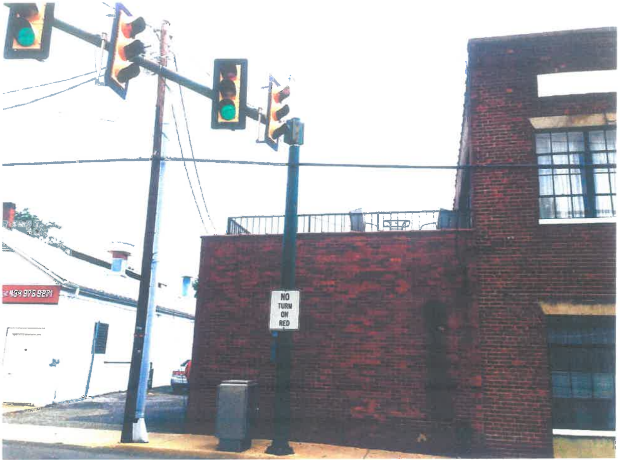
10 TH Street façade showing addition to the north side.
