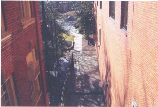
EXISTING VIEW FROM ABOVE LOOKING TOWARDS EAST HIGH STREET
