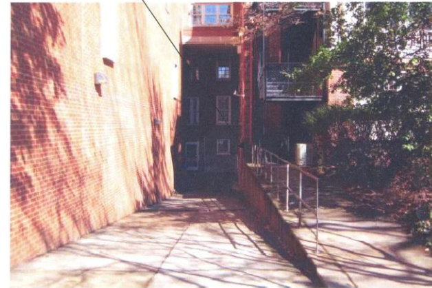
EXISTING VIEW LOOKING DOWN ALLEY BETWEEN PATTERSON AND SOUTH WINGS
