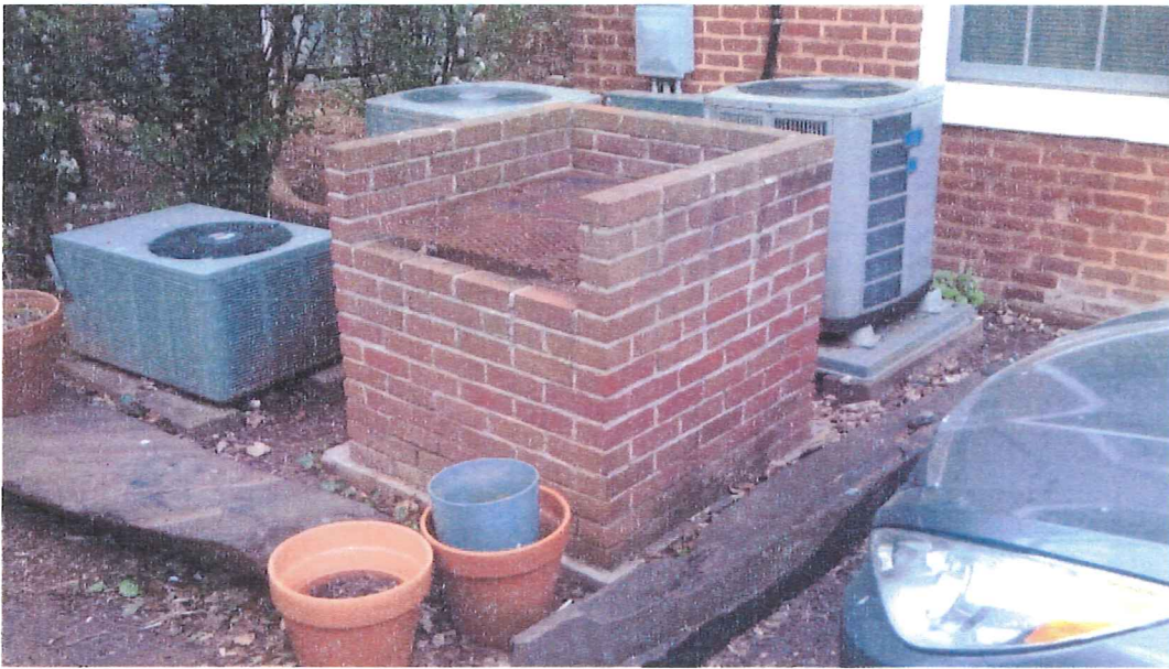
BRICK BARBECUE & BASE TO BE REMOVED AND SOME BRICKS SET INTO DIRT BELOW TO CREATE WALKABLE SURFACE.
