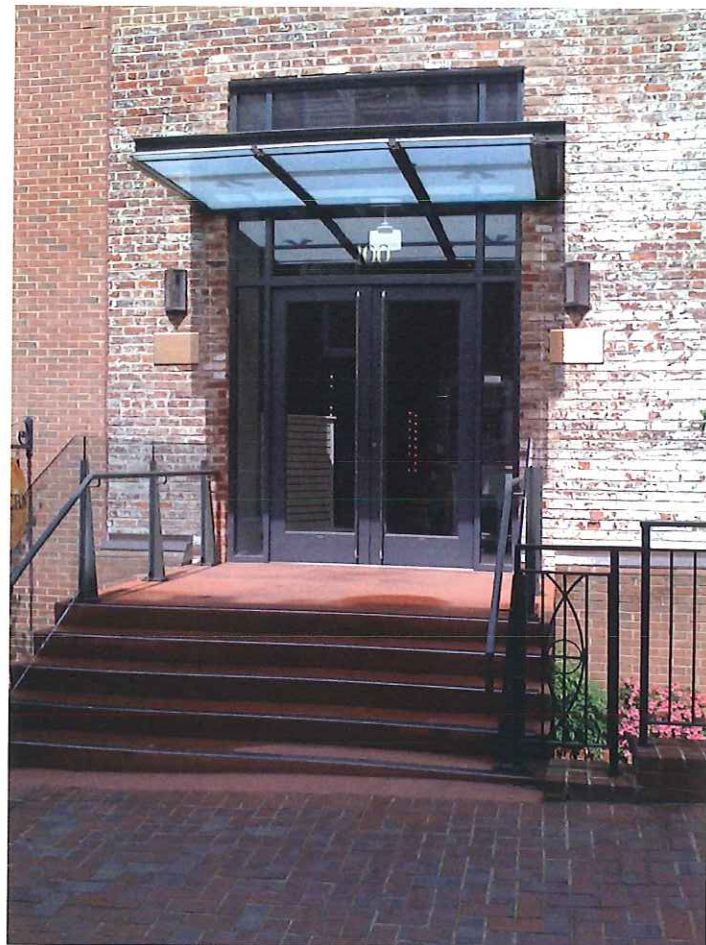
SIDE DOOR AT CASPARI, 1ST ST. S AND MAIN ST.
