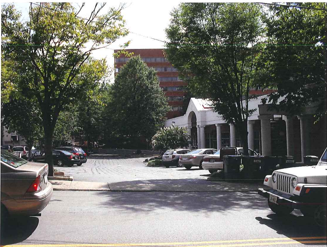
VIEW OF PARKING, EAST, AND NORTH ELEVATIONS FROM WEST MARKET STREET
