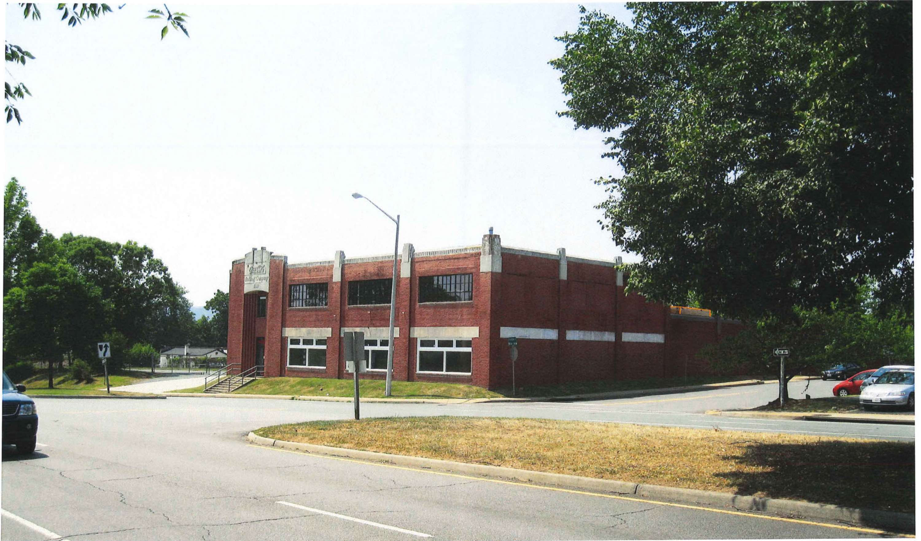
Sight lines: Rooftop mechanical equipment - Preston Avenue
