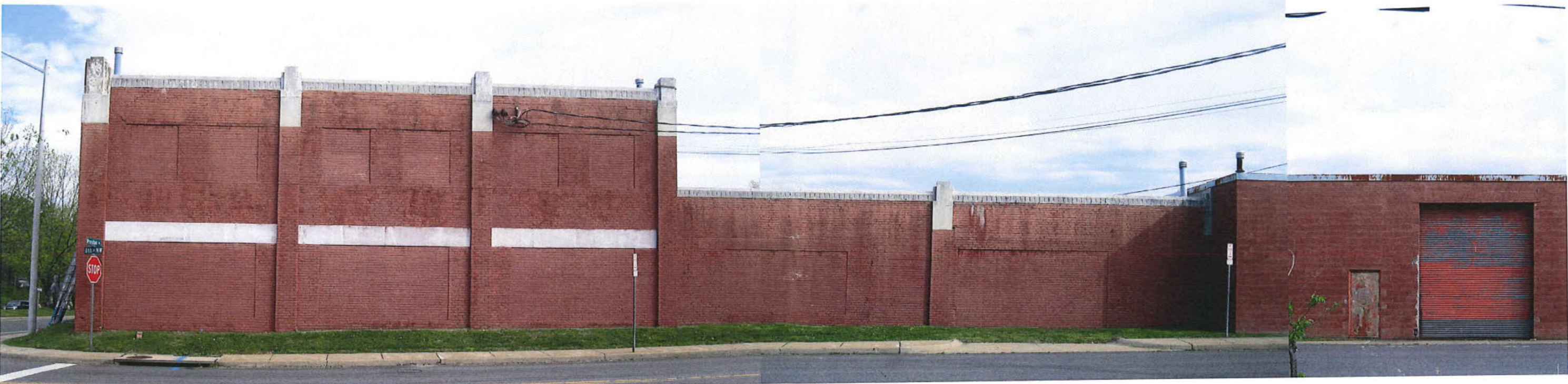
Site photos: Preston Avenue (top), 8th Street (bottom)
