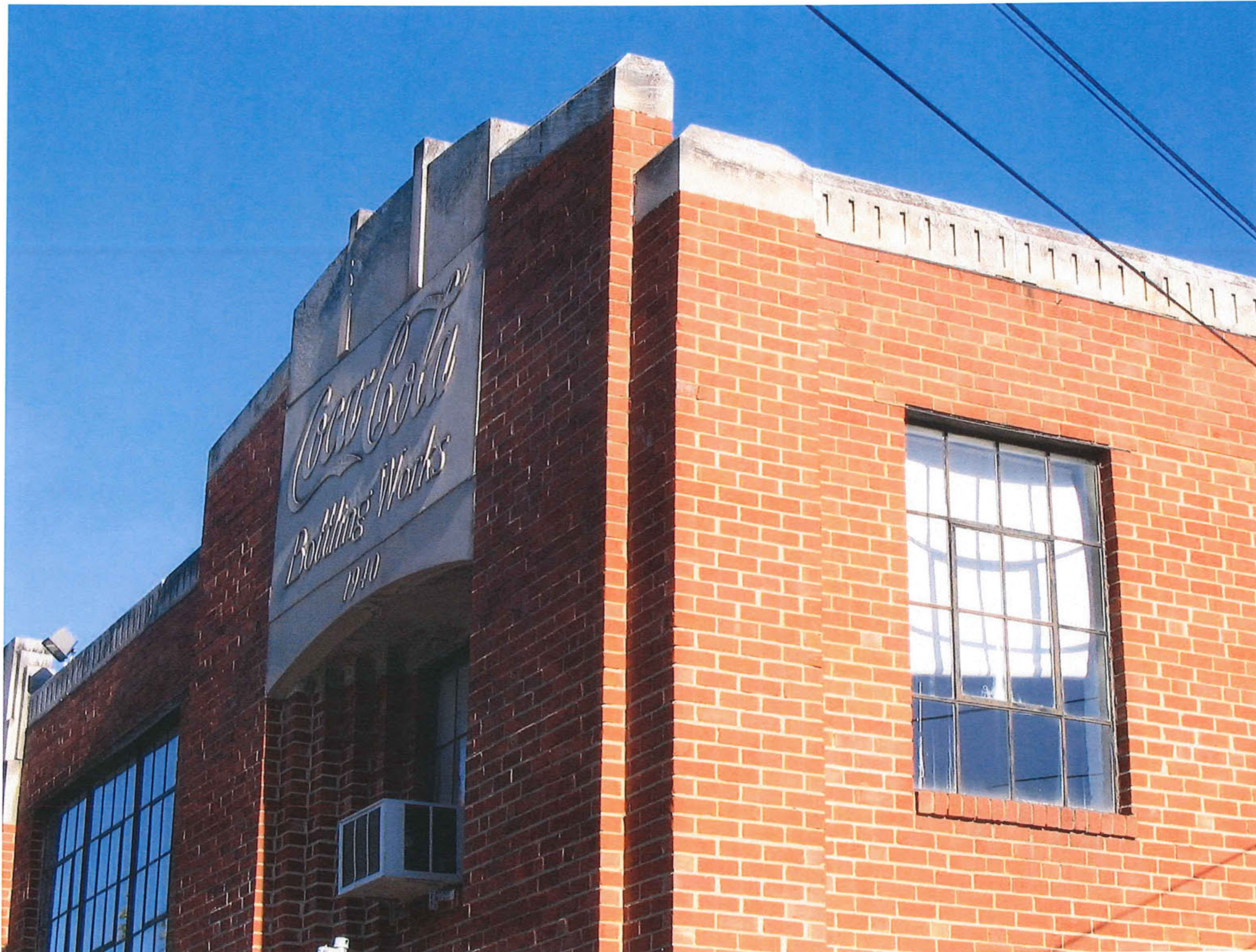
exterior view of awning operators and muntin pattern
