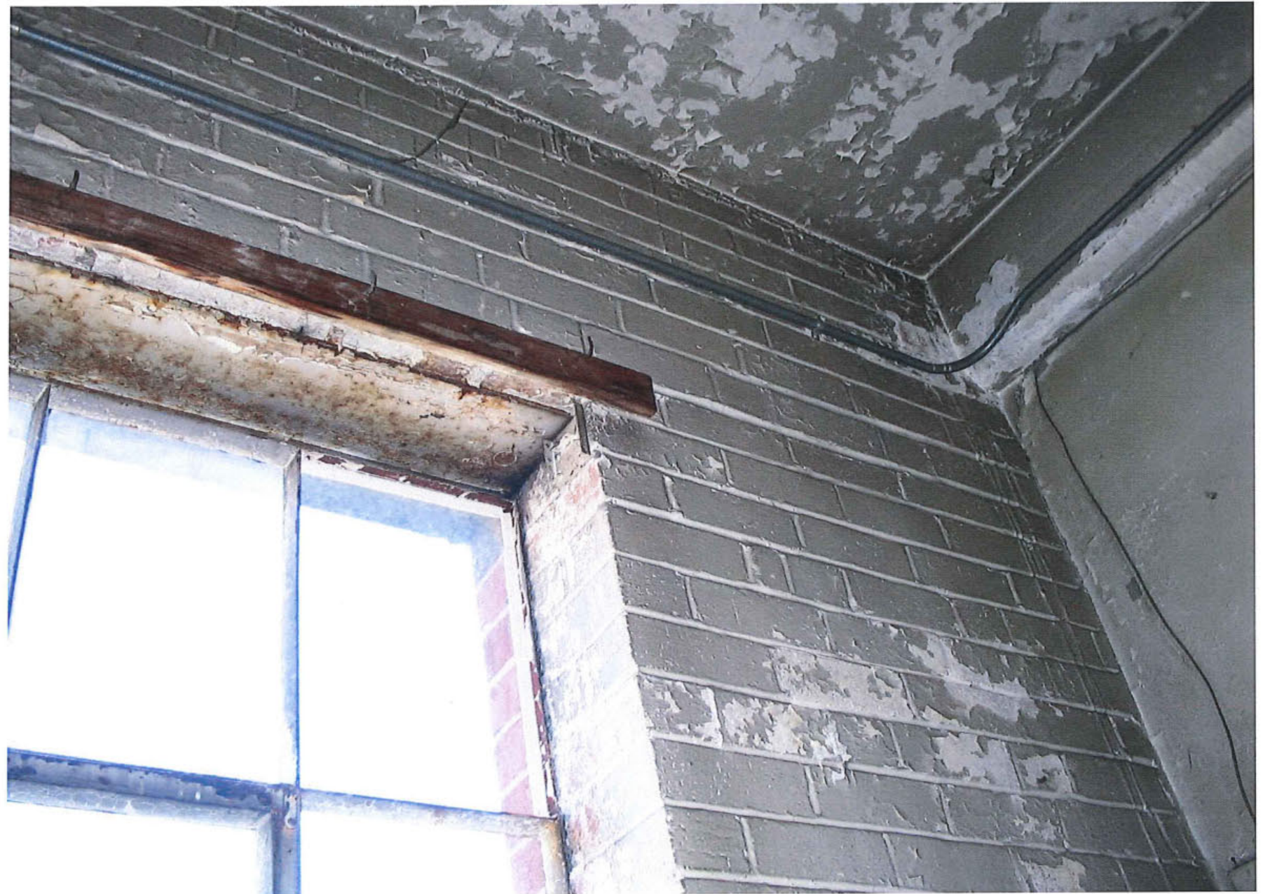
interior photographs of detailing of steel windows, showing interior putty glazing
