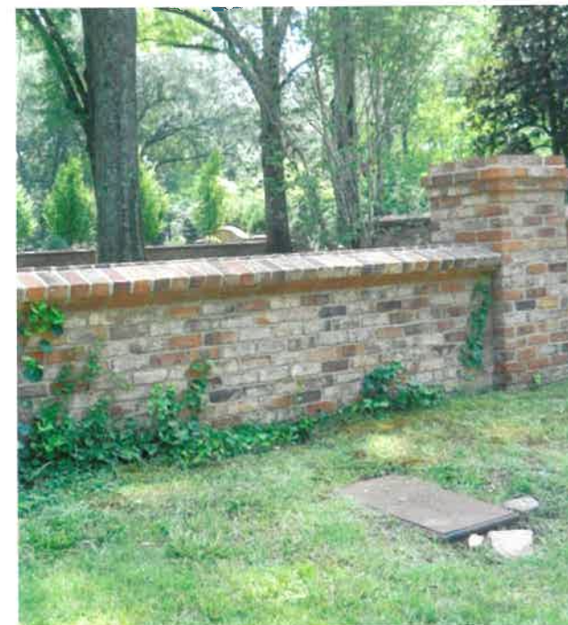
2 Brick retaining walls
