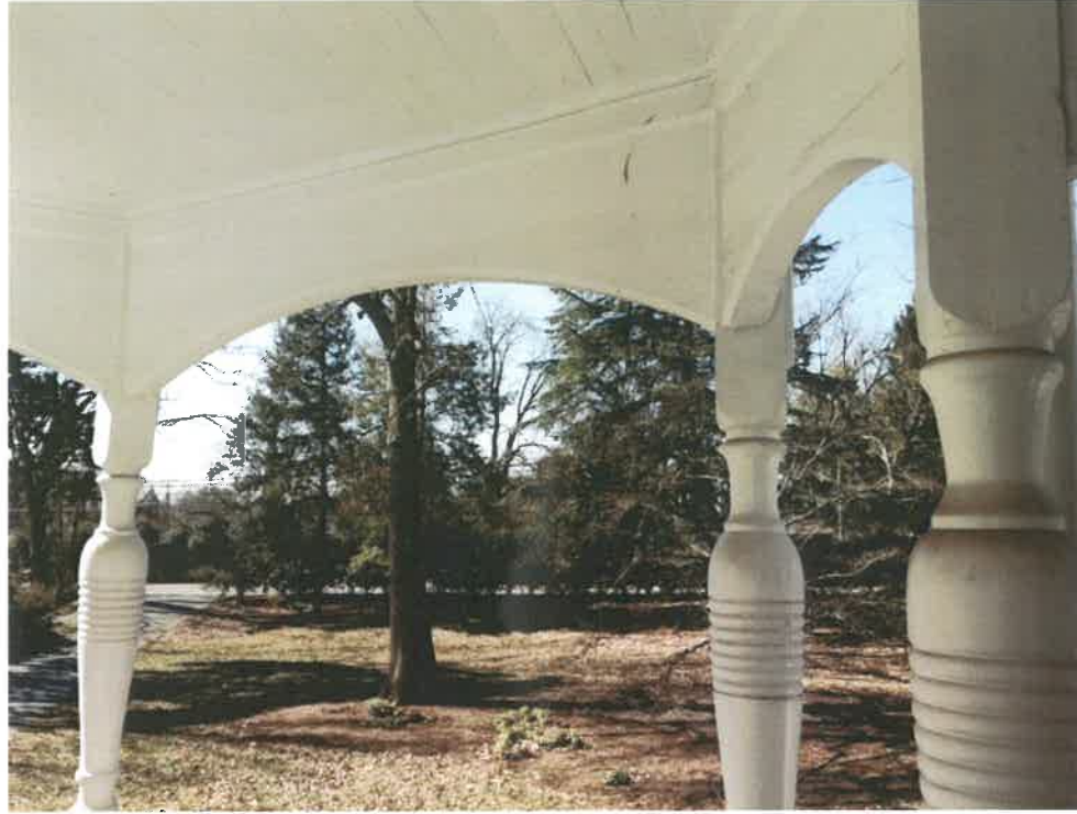
EXISTING PORCH STRUCTURE
