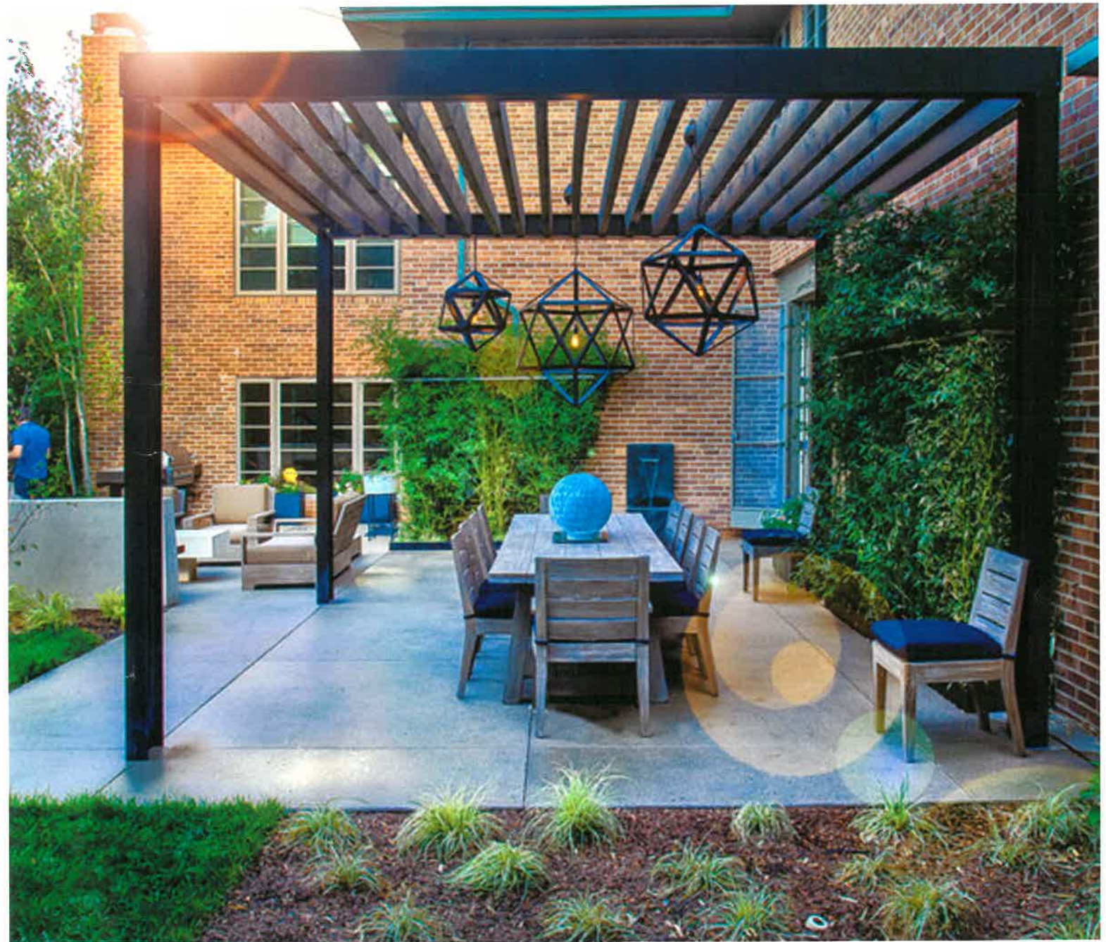
1 Proposed pergola: Steel frame with wooden joists painted black to match existing kitchen addition
