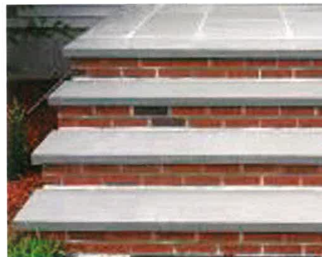
3 Stairs; brick risers with bluestone treads
