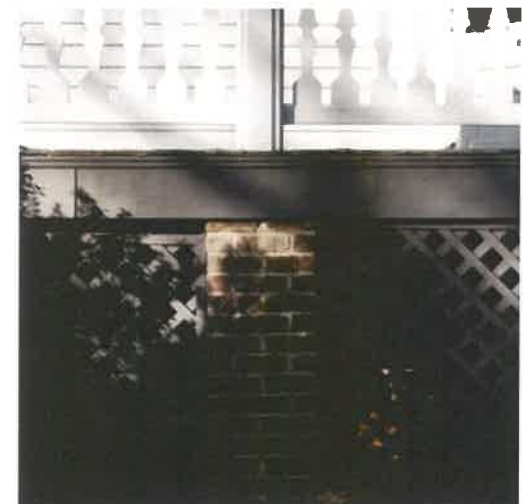
C. EXISTING PORCH STRUCTURE
