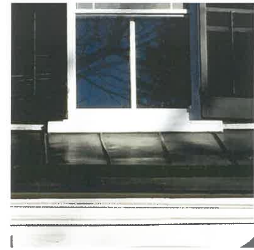
A. ROOF AT WINDOW SILL DETAIL
