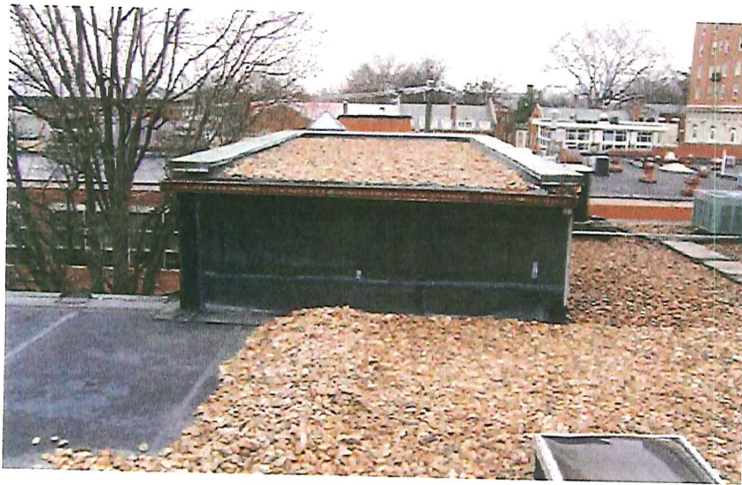
Stairway and elevator roofs are raised above the main section.
