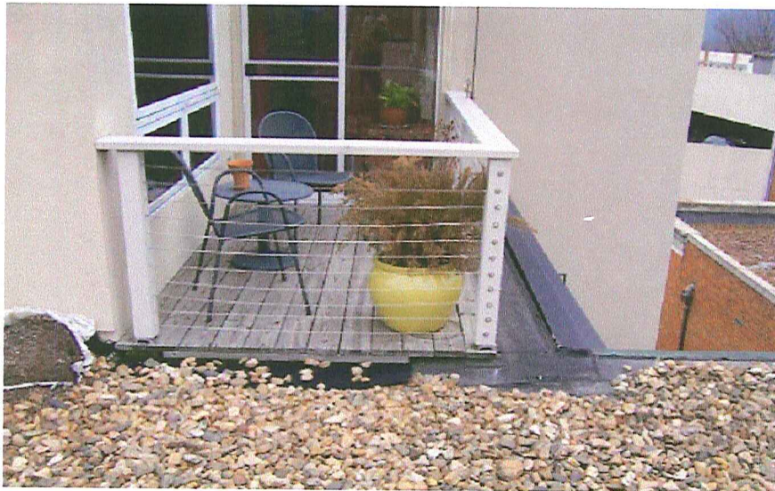
Replacement of wood decking is not included in our budget. Demolition is included since it will be necessary to do so for roof replacement.
