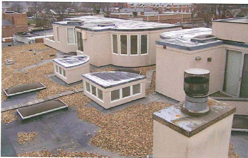
Overview of south roof area.
