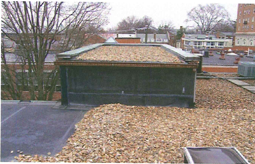
Stairway and elevator roofs are raised above the main section.
