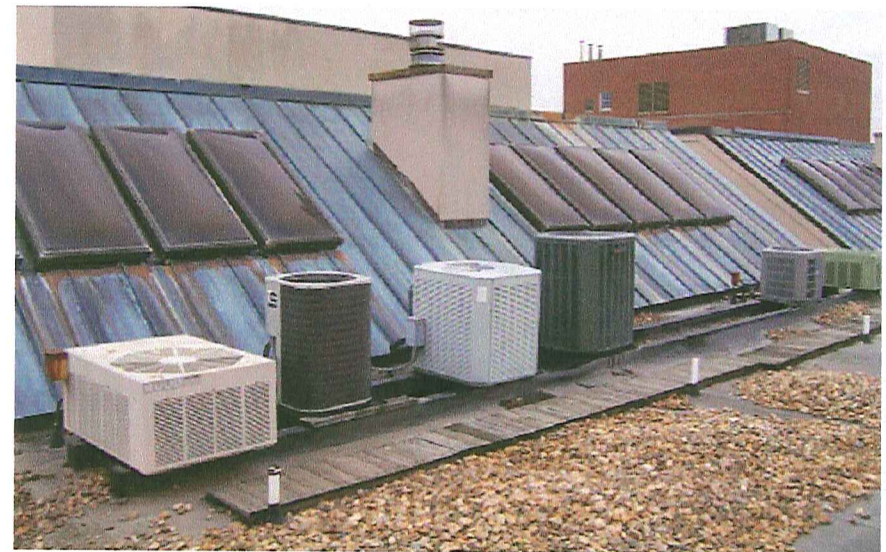
The sleeper rails that support the heat pumps need to be removed and replaced in a new position that doesn't block water from the copper roofs.
