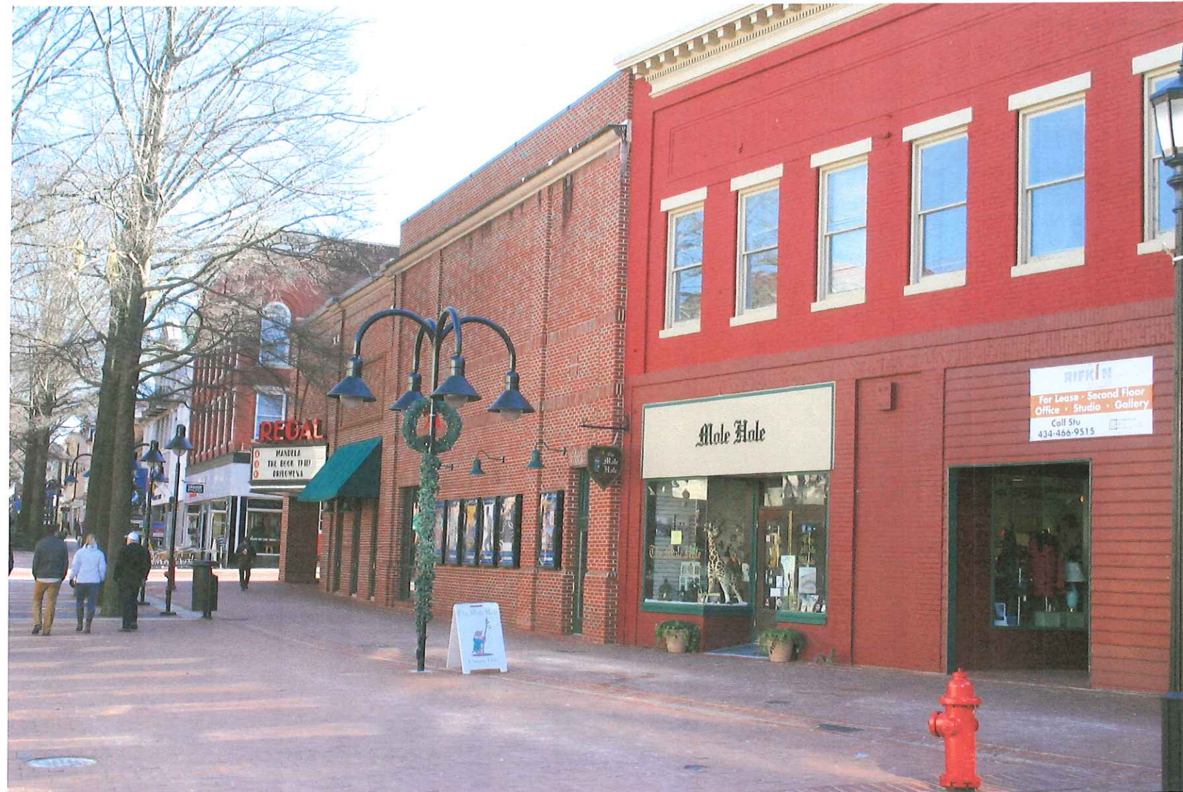
7. Current photograph- existing conditions showing building just to the west of property.
