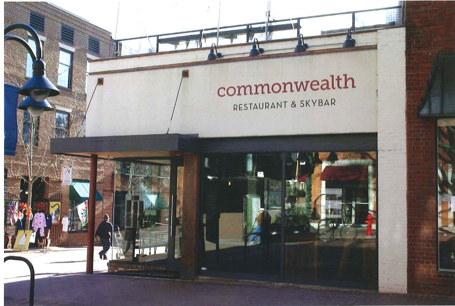
5. Current Photograph Commonwealth Restaurant Modern architecture, exposed structural steel elements, large glass openings, patinated metal panels.
