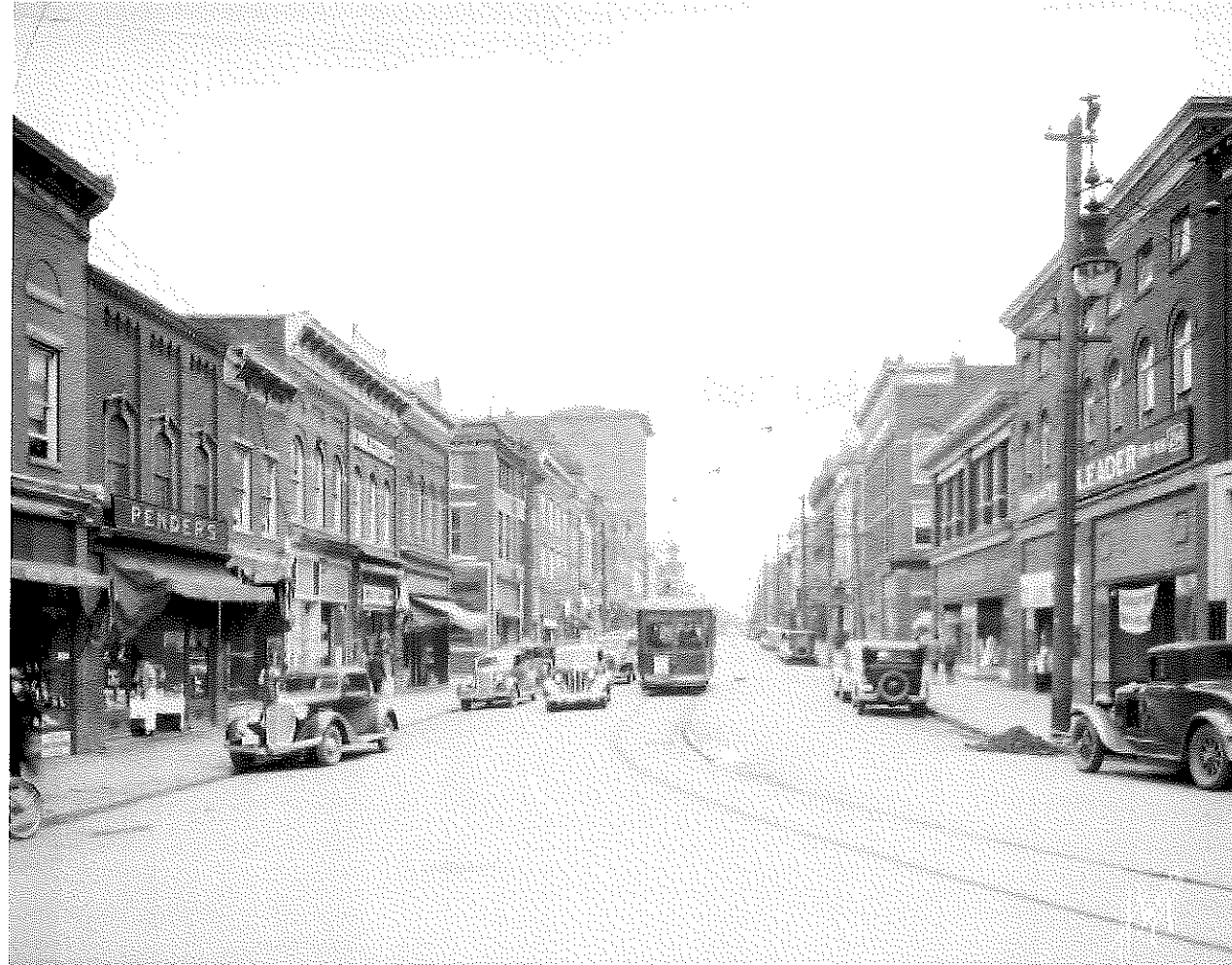
5. Historic photo circa 1930's Property appears at right. Condition prior to first Legget and Sears.
