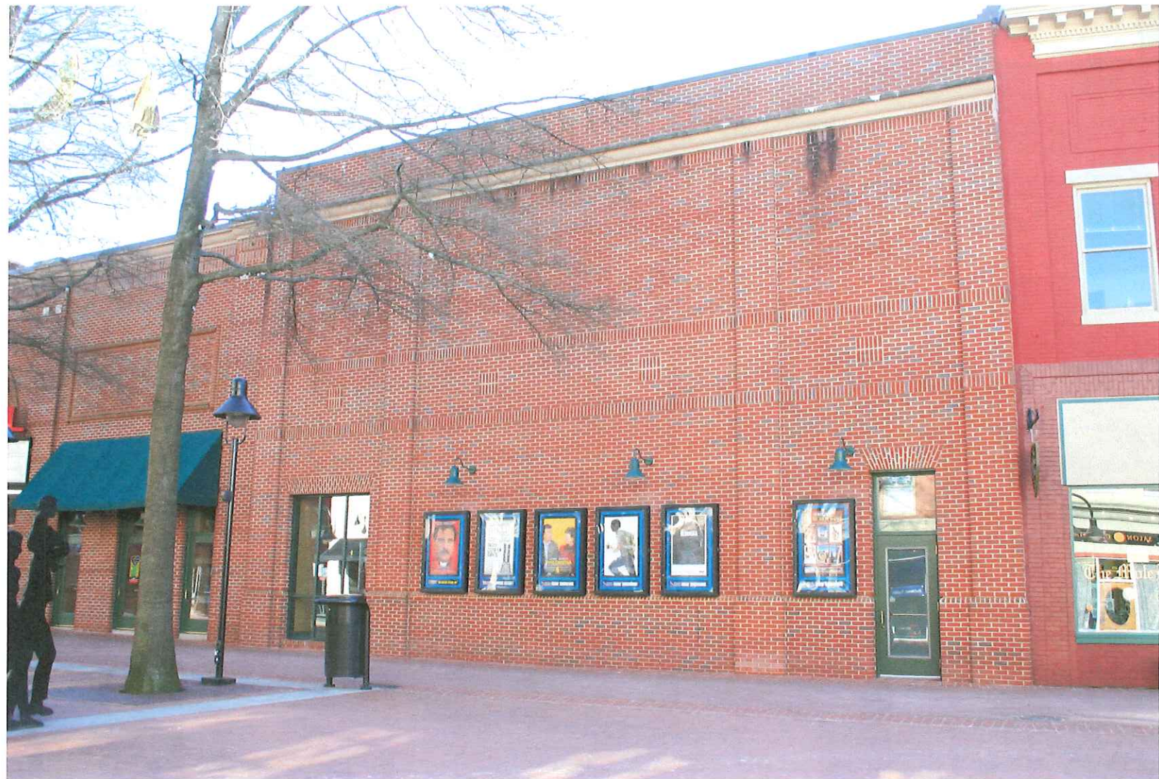
2. Current photograph- existing conditions.
