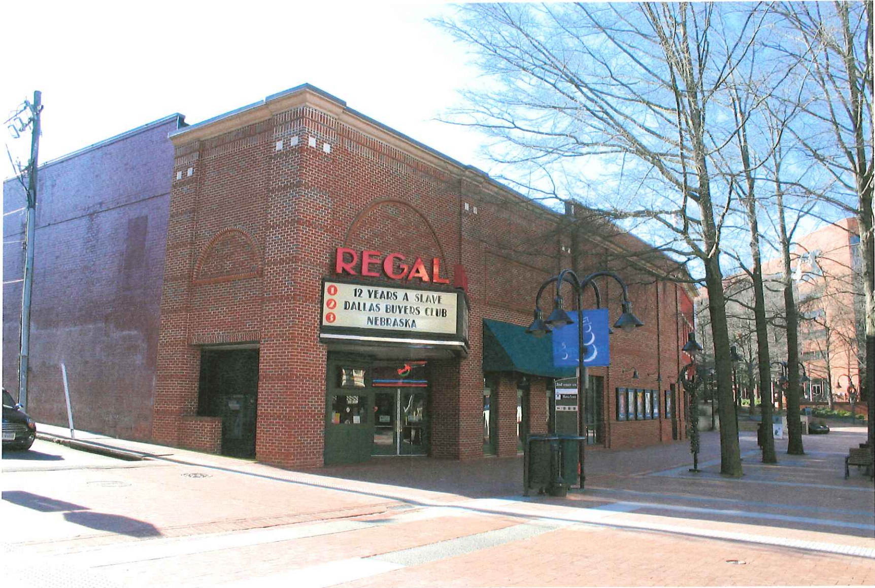
1. Current photograph- existing conditions.
