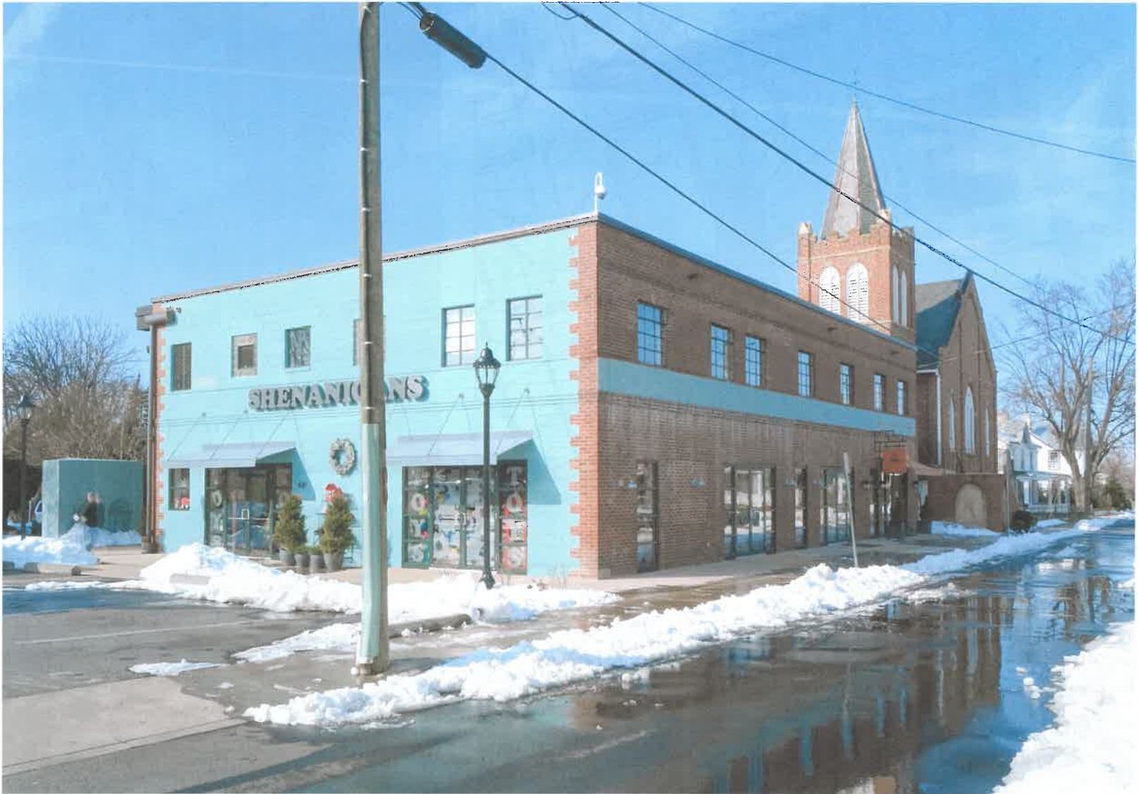
VIEW OF EXISTING BUILDING LOOKING NORTH FROM WEST MAIN STREET AREA
