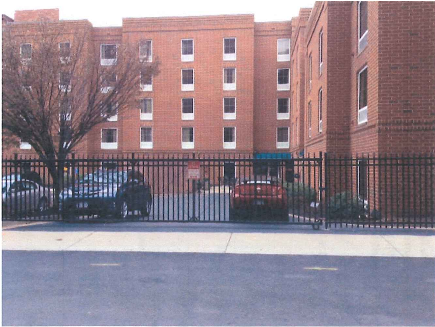
< View of site from 9th street between Hampton Inn and The Flats @ West Village.
