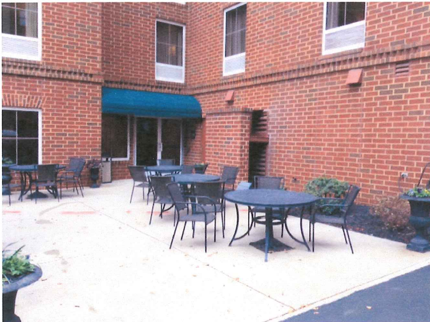
< Existing patio to be replaced with pervious pavers. Existing laundry vent enclosure to be roofed.
