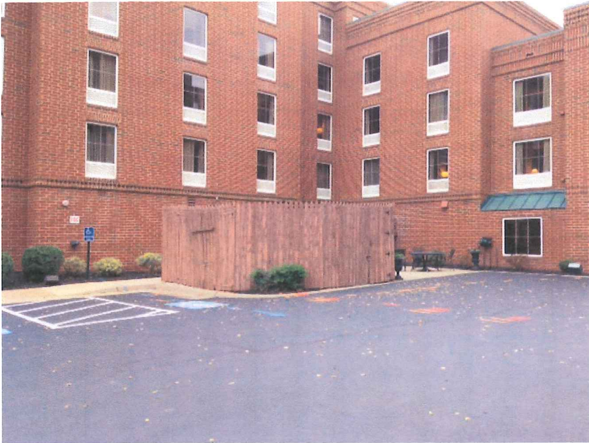
< Existing wood generator enclosure and existing patio.
