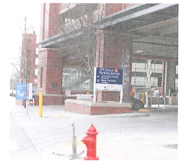
UVA | PARKING GARAGE, 117 11TH ST SW
