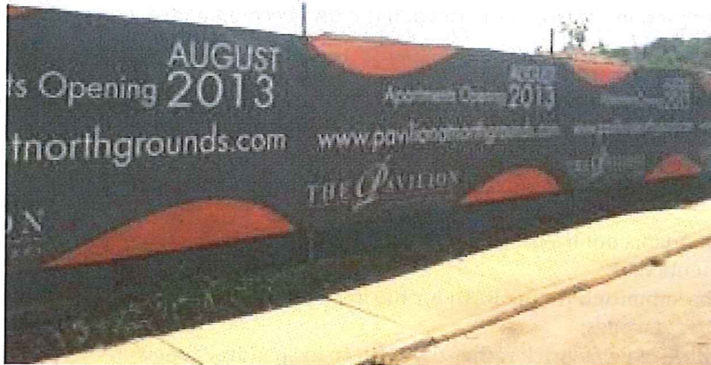
an example of fence wrap used at the Pavilion at North Grounds while under construction
