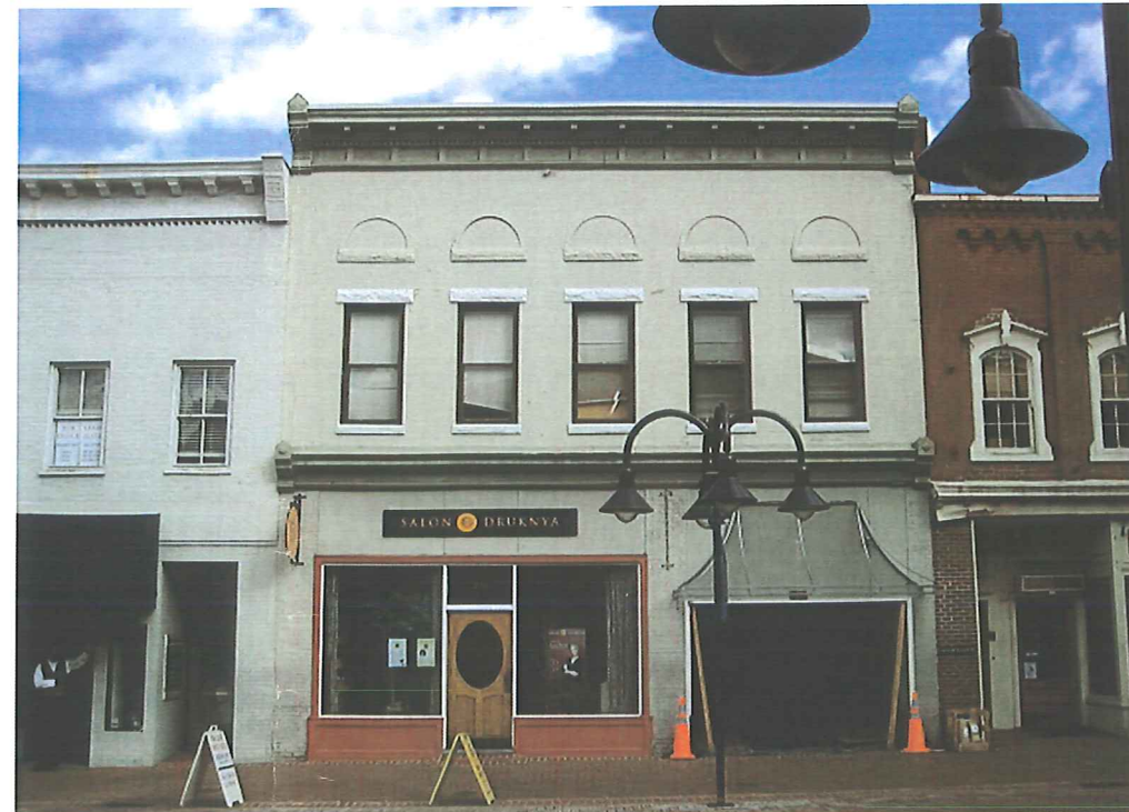
Image of Full Building Elevation @ 219 West Main Street
