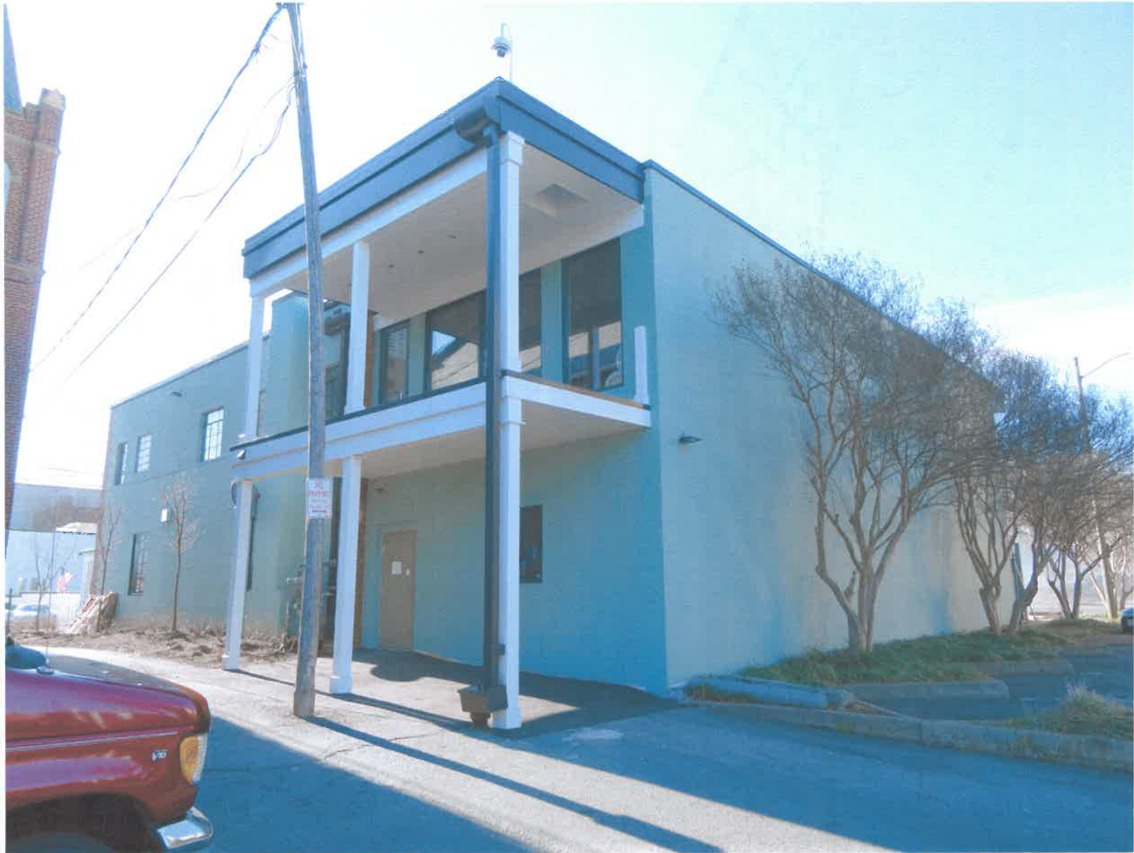
VIEW LOOKING SOUTH EAST FROM WEST PARKING AREA - PHOTO
