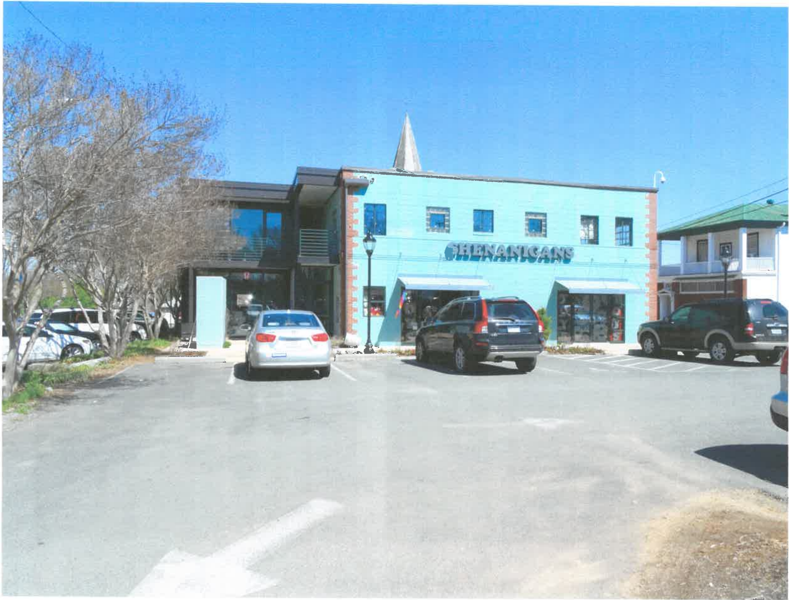
VIEW OF EXISTING BUILDING LOOKING NORTH FROM WEST MAIN STREET AREA
