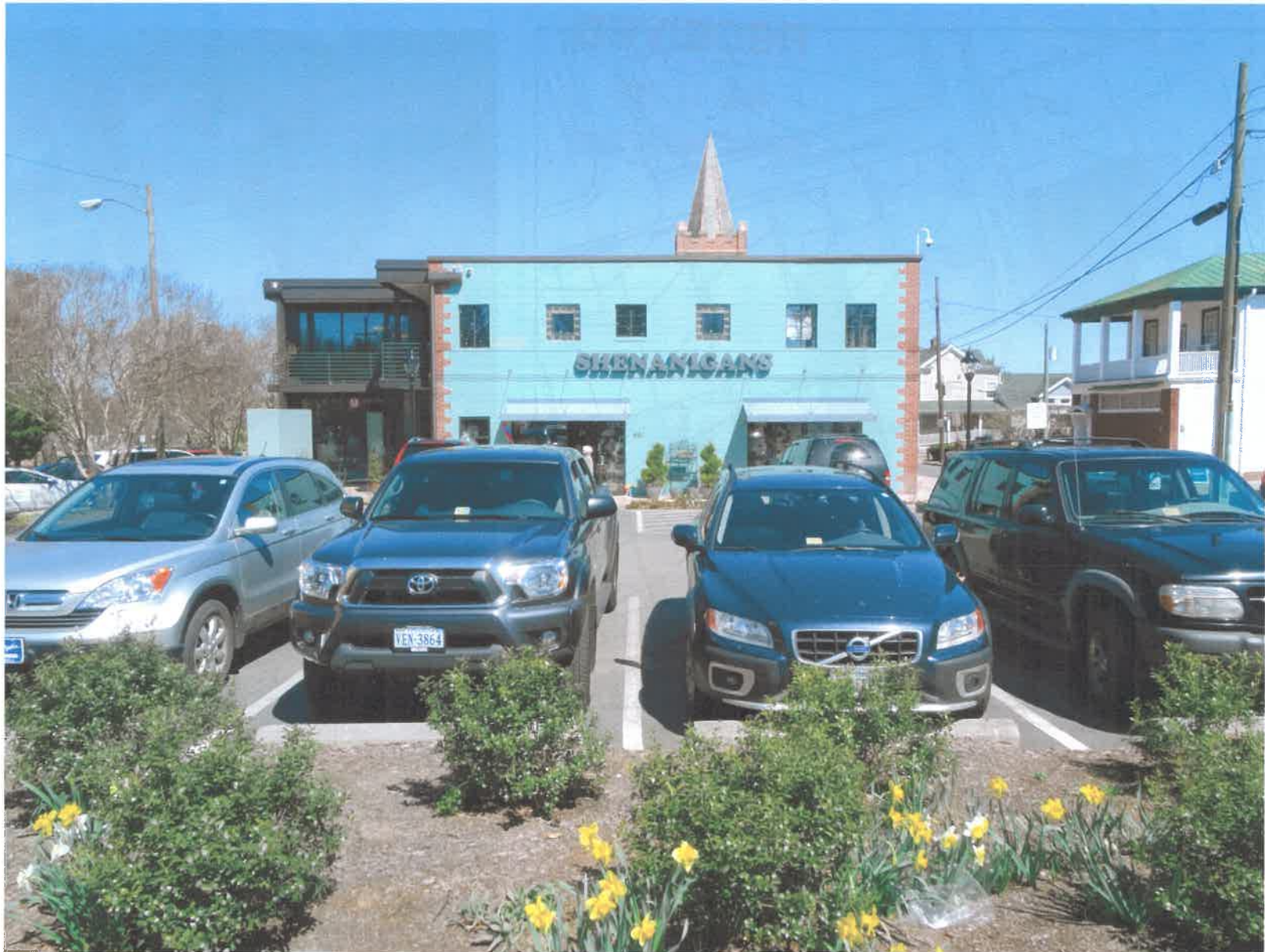
VIEW OF EXISTING BUILDING LOOKING NORTH FROM WEST MAIN STREET AREA
