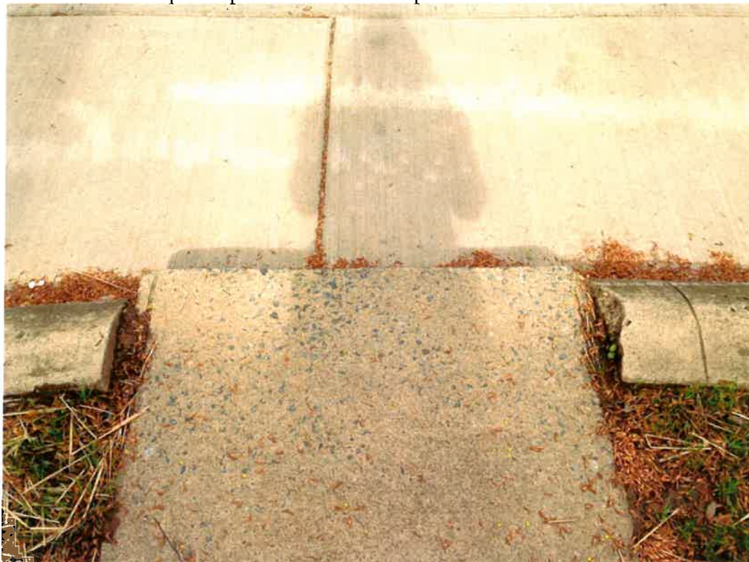
This existing sidewalk extends beyond the concrete curb into the City sidewalk so removal of the sidewalk would require replacement of at least part of the curb.
