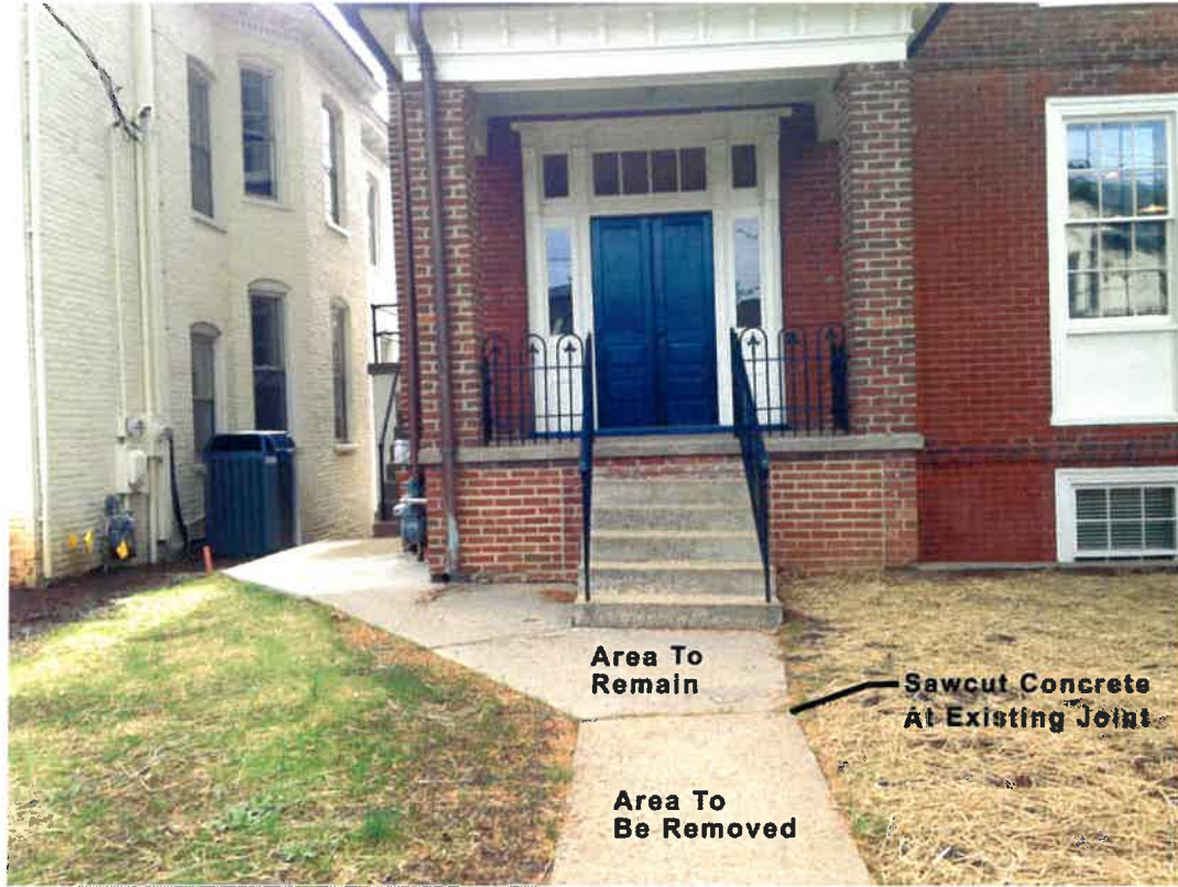
This existing sidewalk extends beyond the concrete curb into the City sidewalk so removal of the sidewalk would require replacement of at least part of the curb.
