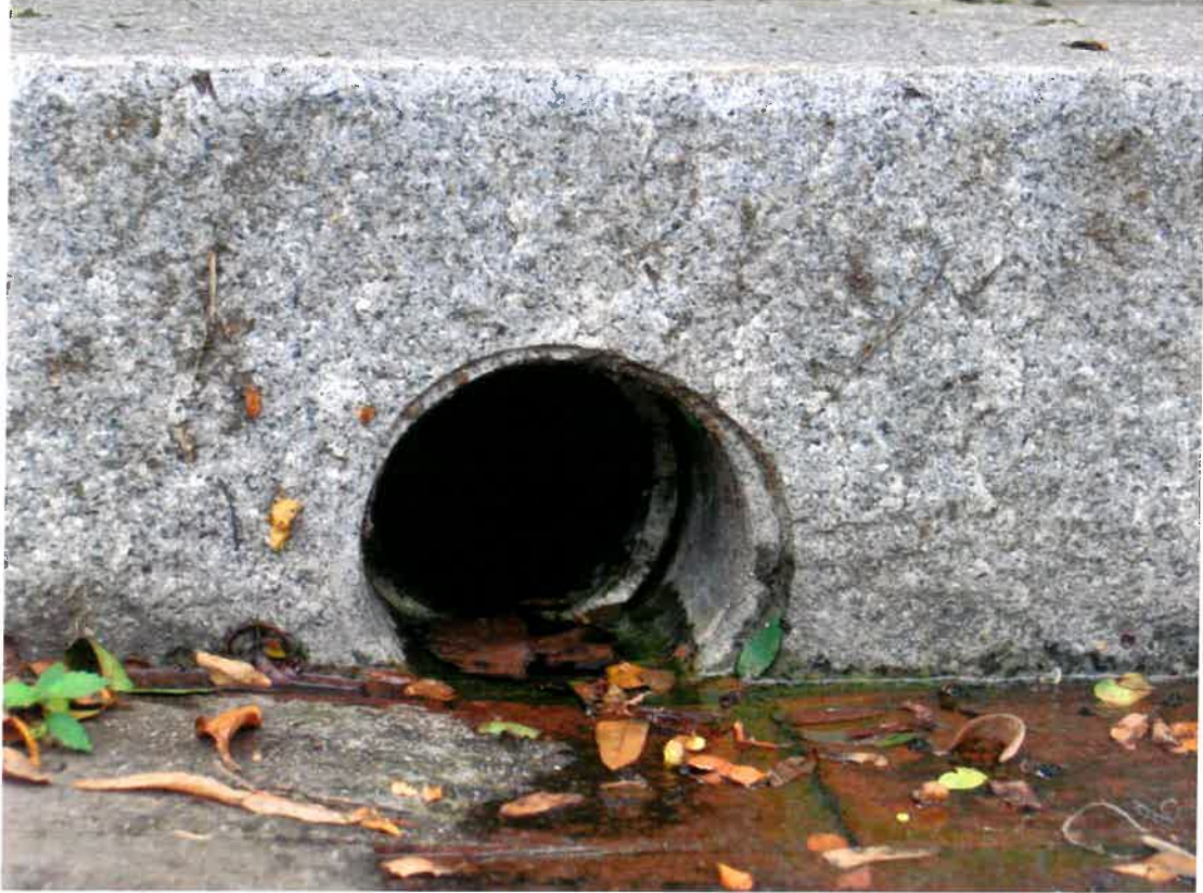
Existing drain pipe through granite curb.
