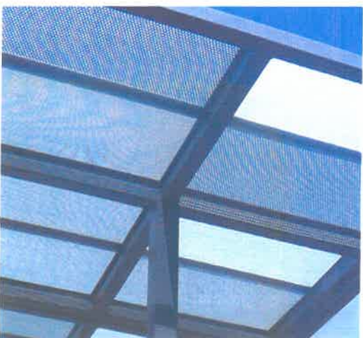
ROOF CANOPY -PERFORATED STEEL
