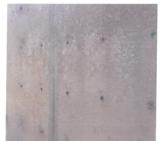
FOUNDATION - EXPOSED CAST IN PLACE CONCRETE
