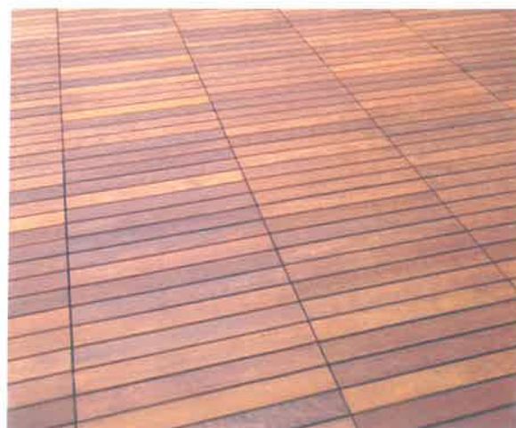
ROOF TERRACE -IPE DECK PANELS
