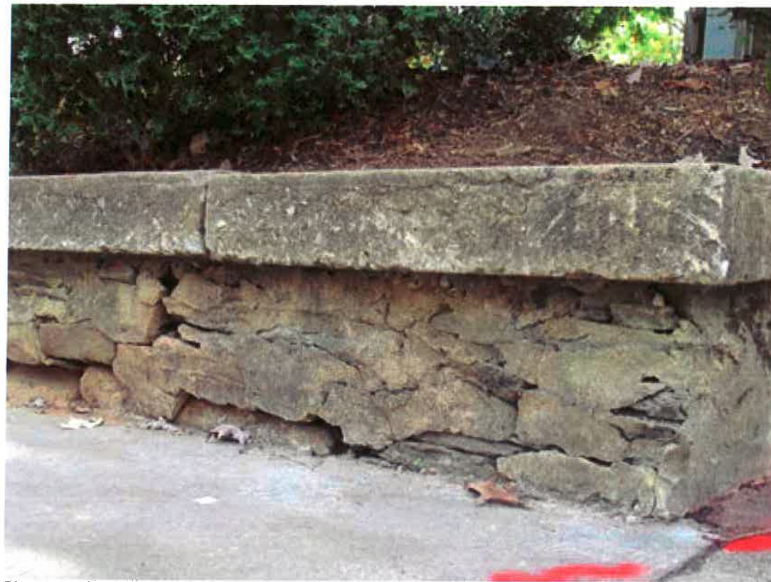
Photograph 4 - Parge Coating along East Elevation near 2nd Street Stairway
