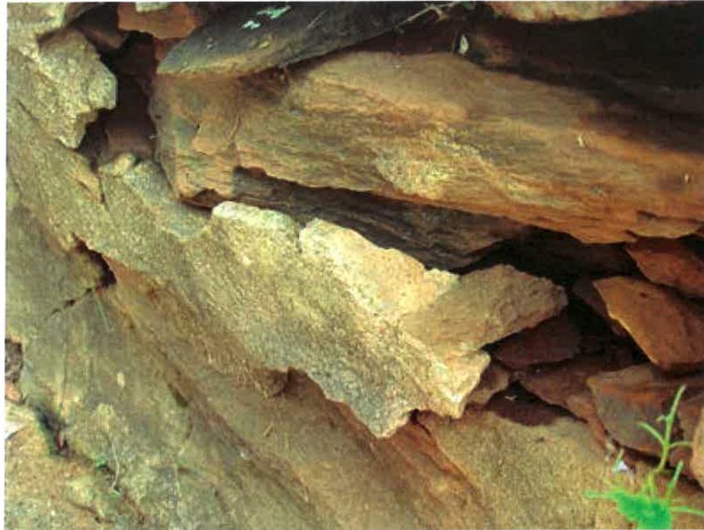
Photograph 10 - Stacked Stone + Parge Coating
