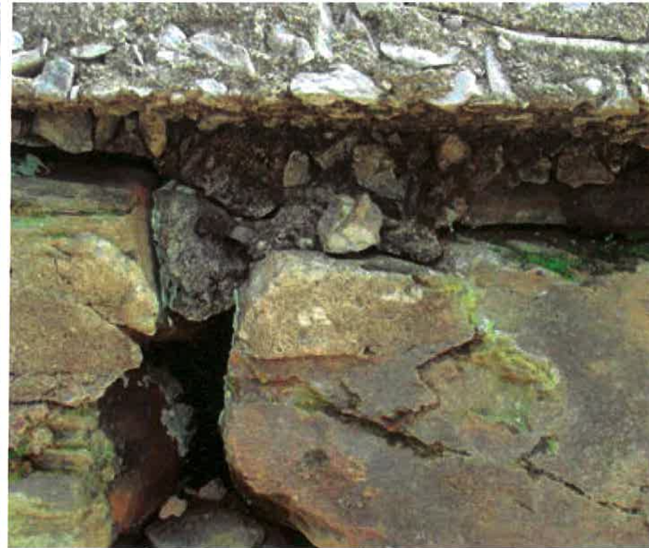
Photograph 13 - Concrete Cap Cast Atop of Stone Wall
