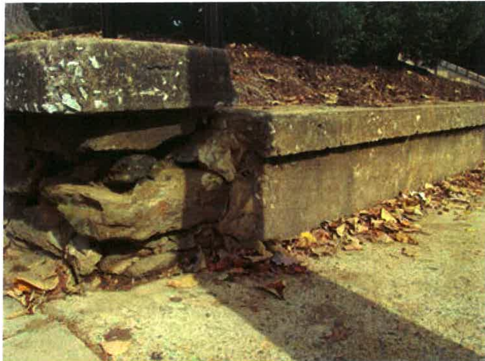
Photograph 18 - Concrete Wall with Integral Concrete Cap
