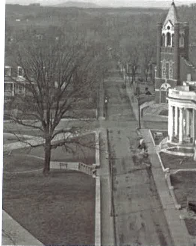
Plate 2 Enlargement - Note: No Handrails at Stairs
