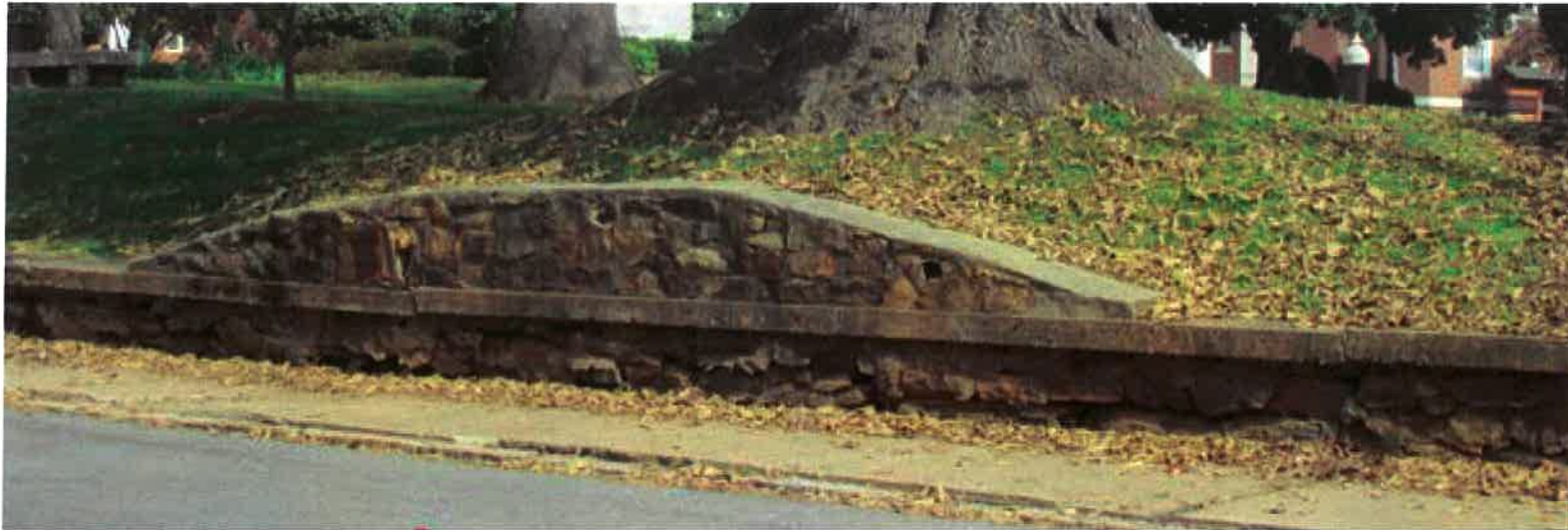
Photograph 16 - Retaining Wall Extension at the American Linden Tree
