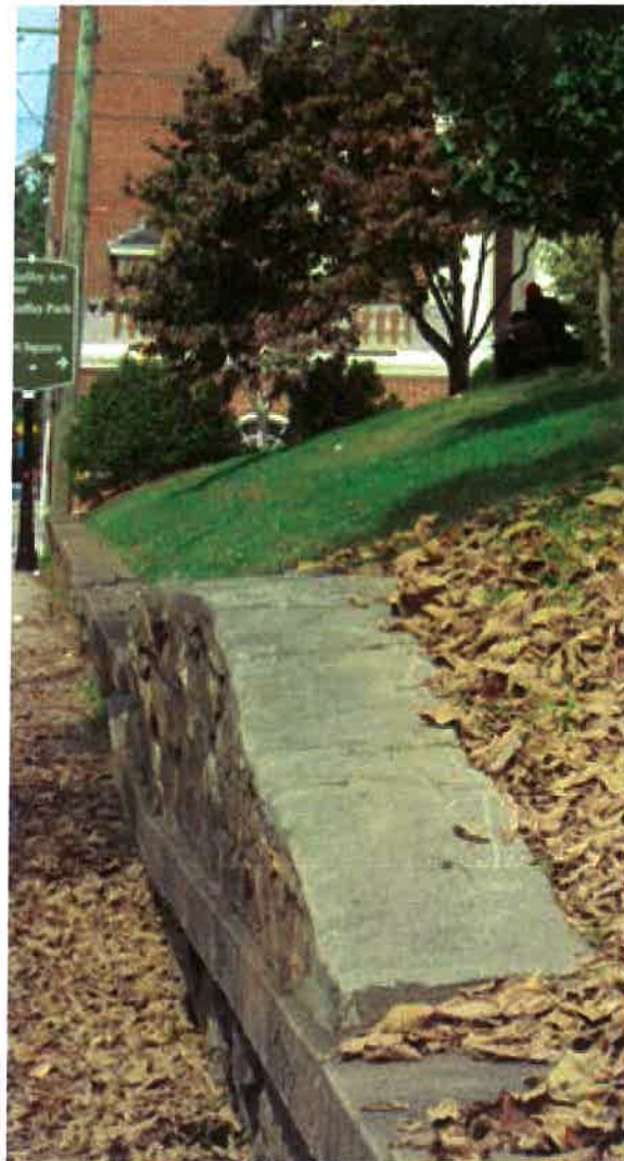
Photograph 17 - Retaining Wall Extension
