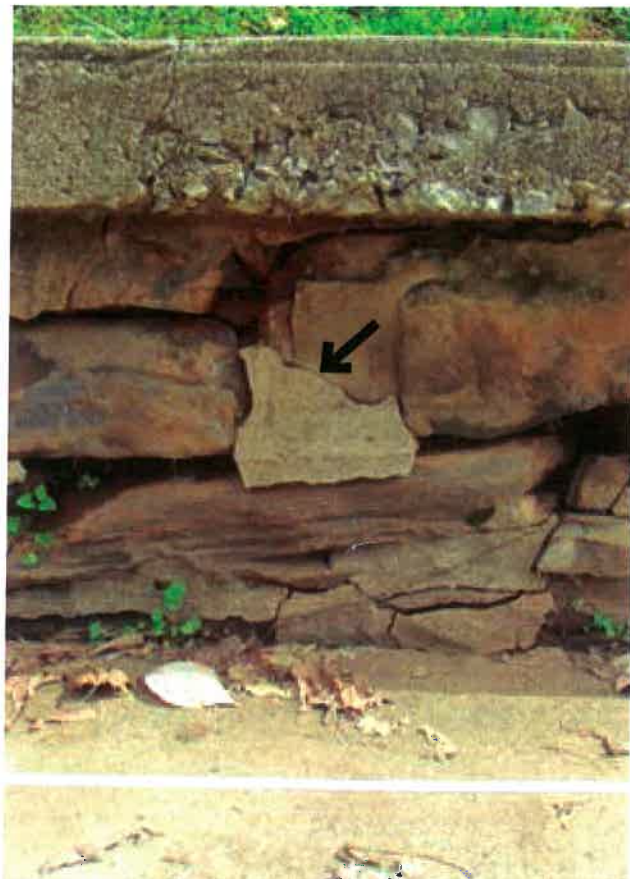
Photograph 9 - Existing Wall (Remnant Parging)
