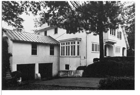
The walls are solid brick with stucco, the roof is metal, tin; heat is provided by gas and hot water.
