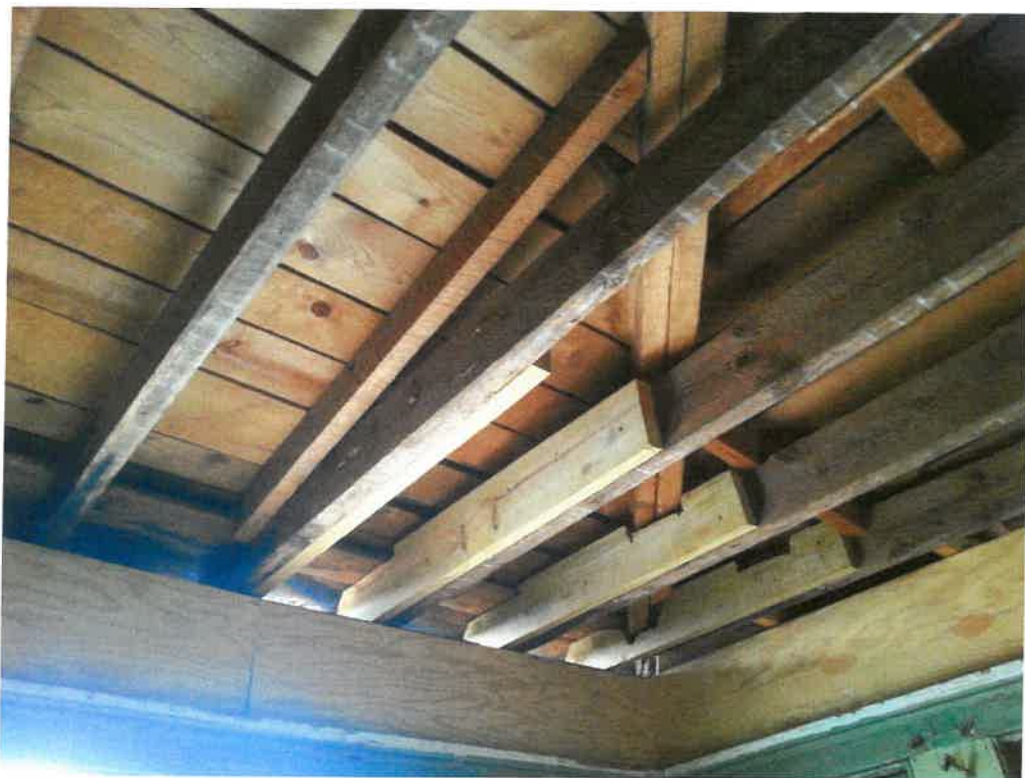
Photo 1 - Partially completed back roof repairs
