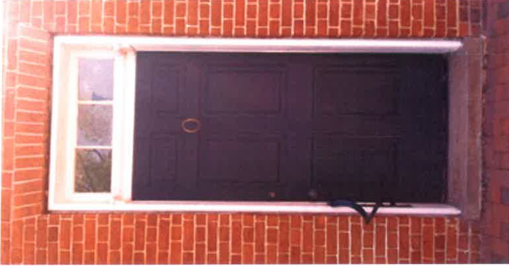
Example of door with narrow brick mold and a transom. Court Square.
