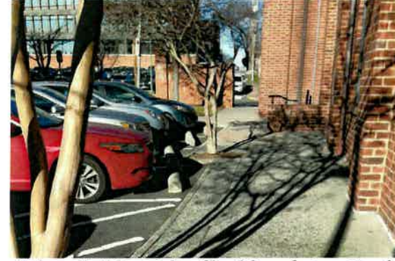
Sidewalk, West side of building facing North
