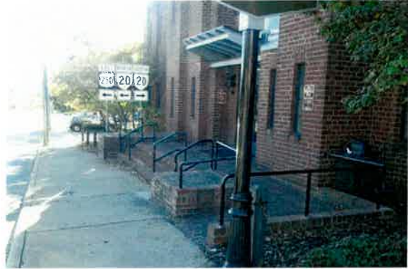
Front steps and ramp facing East
