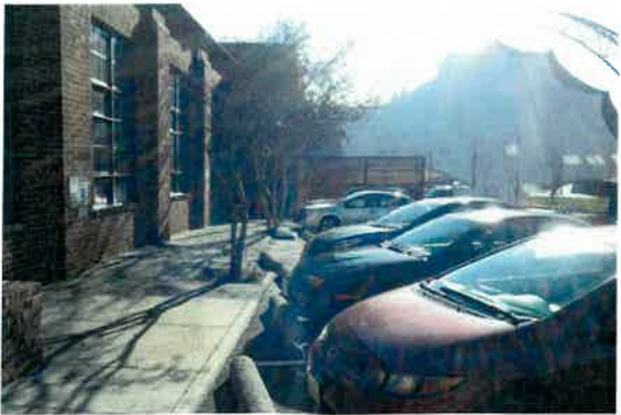
Sidewalk, West side of building facing South
