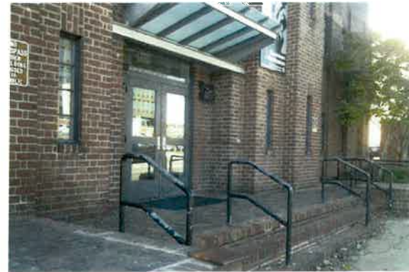
Front steps facing West
