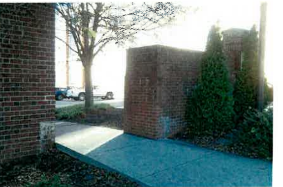
Walkway into West lot
