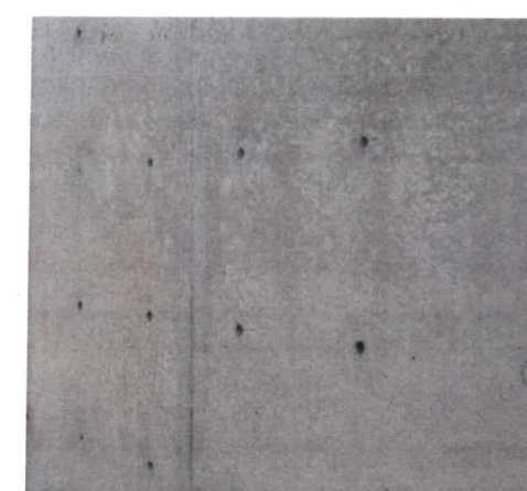
FOUNDATION - EXPOSED CAST IN PLACE CONCRETE
