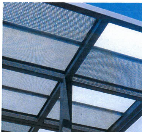
ROOF CANOPY -PERFORATED STEEL
