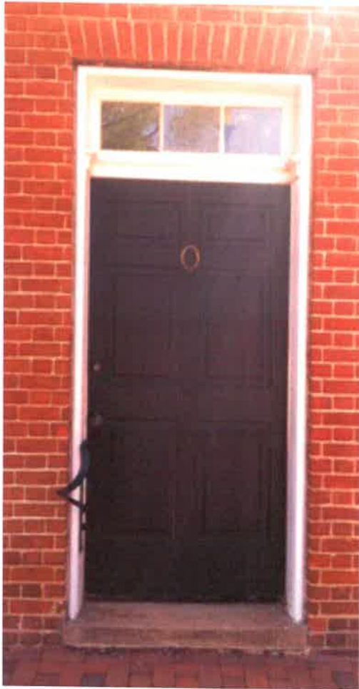
Example of door with narrow brick mold and a transom. Court Square.
