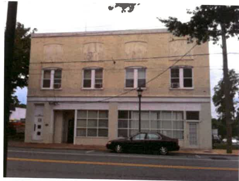
Contiguous property: former Standard Produce Building. Owned by First Baptist Church.
