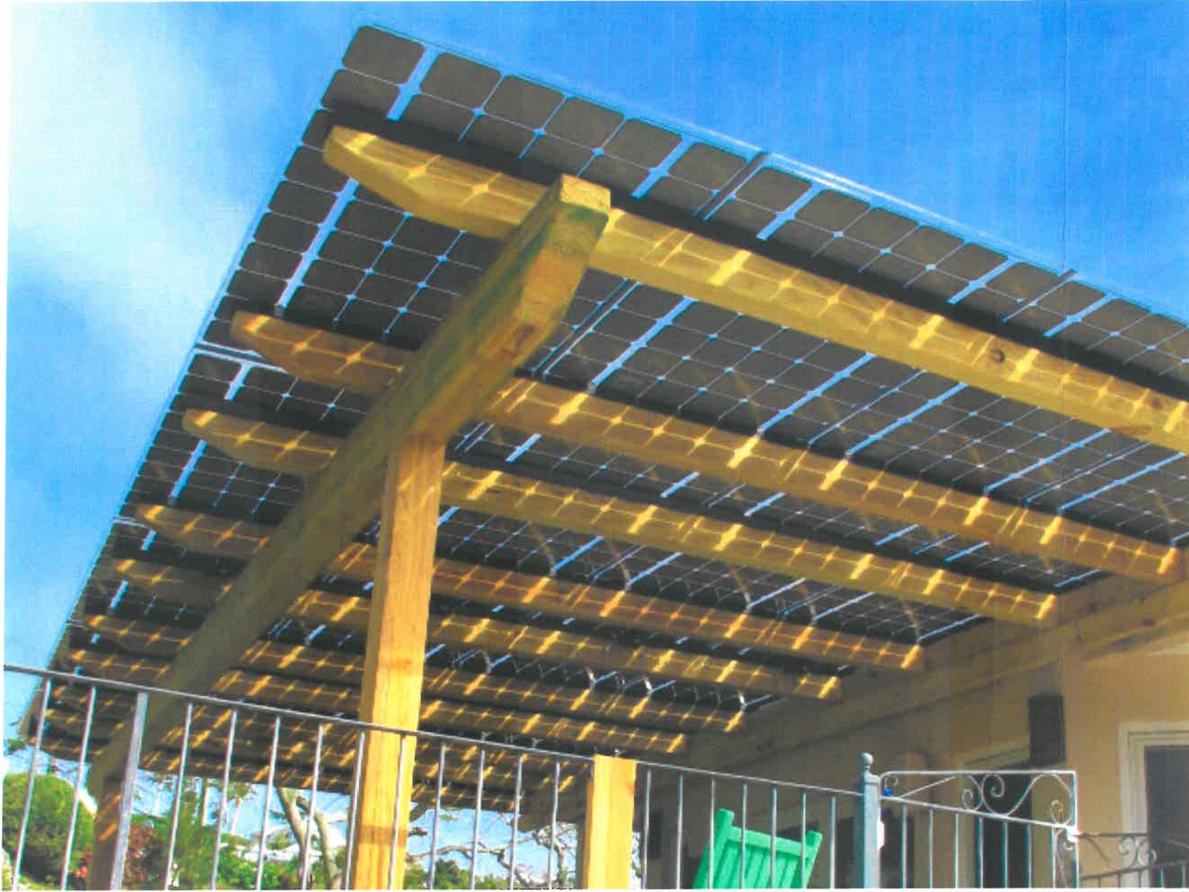
Photo of trellis installation
