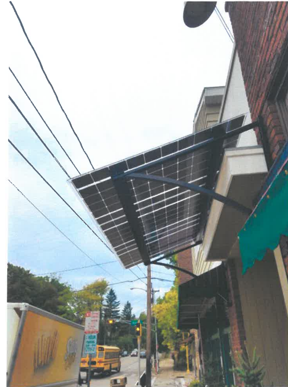
Photo of awning installation
