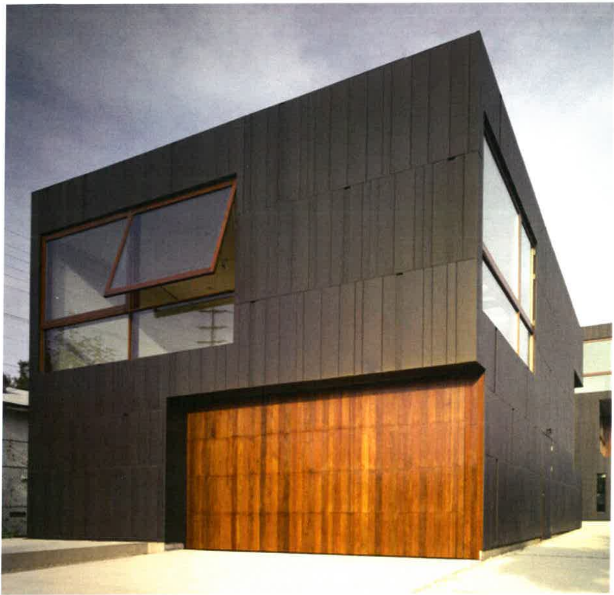
ZINC PANELS - VERTICAL STAGGERED PATTERN
